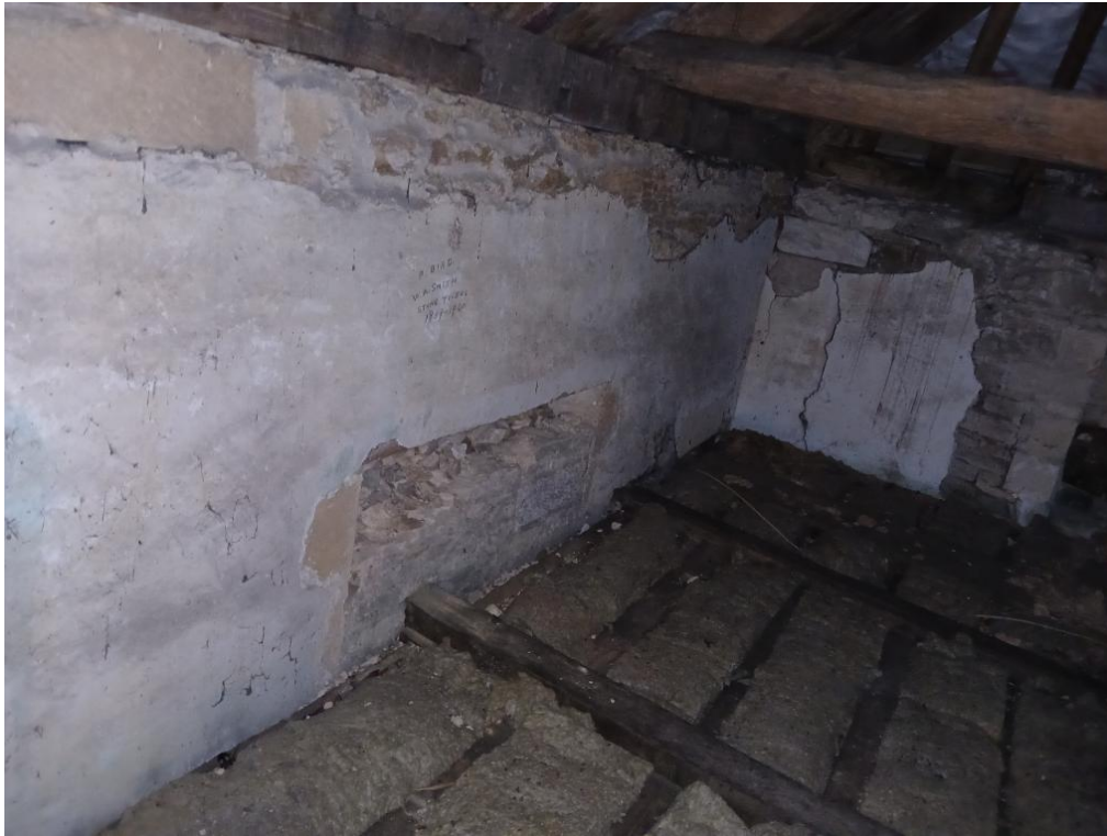
Figure 2 - Filled in window at current ceiling height and previous ceiling joist sockets in wall plate above
