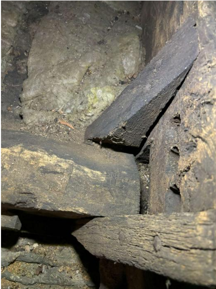
Figure 4 - Typical joint between primary and secondary beams
