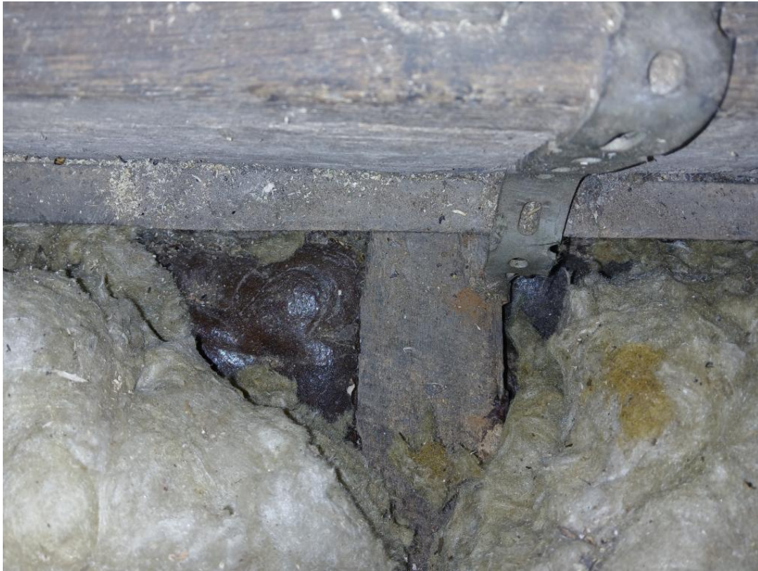
Figure 3 - Joist straps and resin repairs to ceiling
