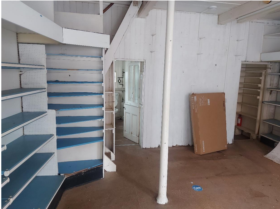
Figure 8: Internal view of rear of former shop
