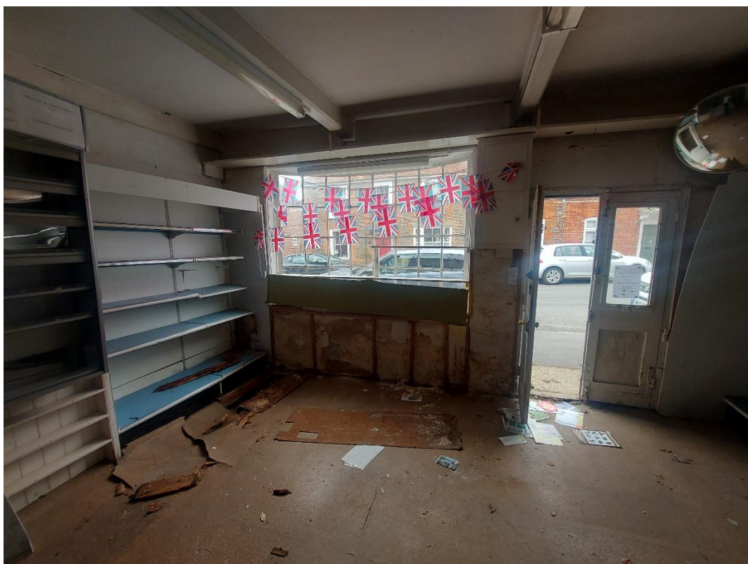
Figure 7: Internal view of former shop
