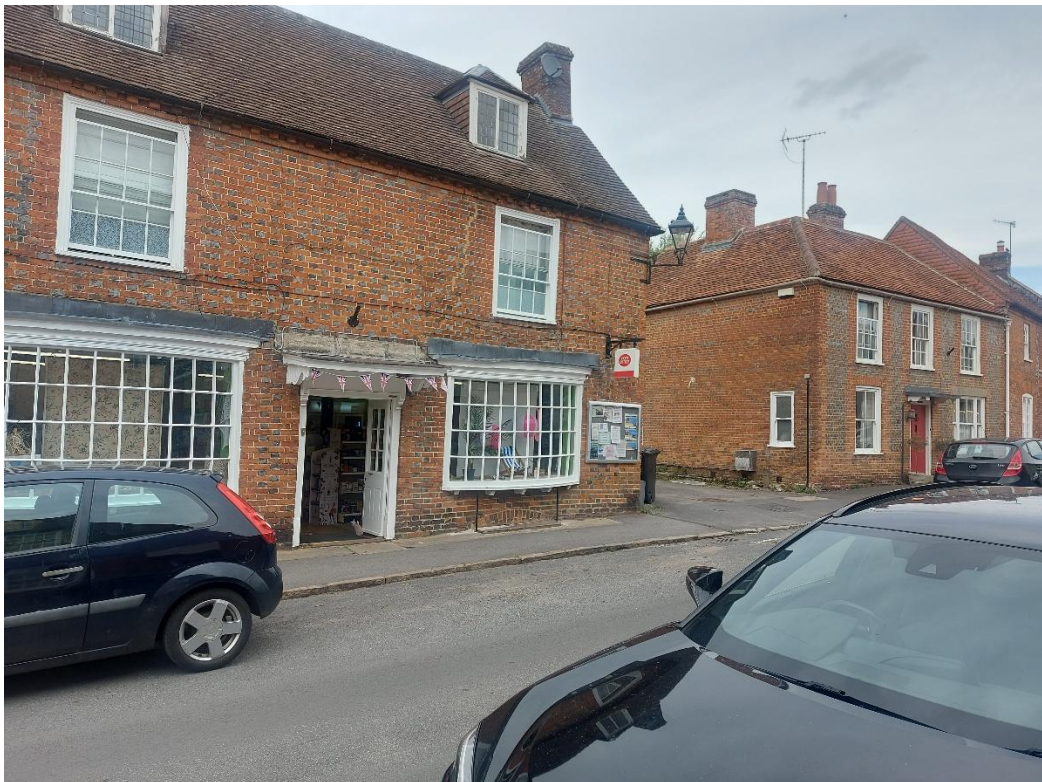
Figure 3: Post office at 6 High Street
