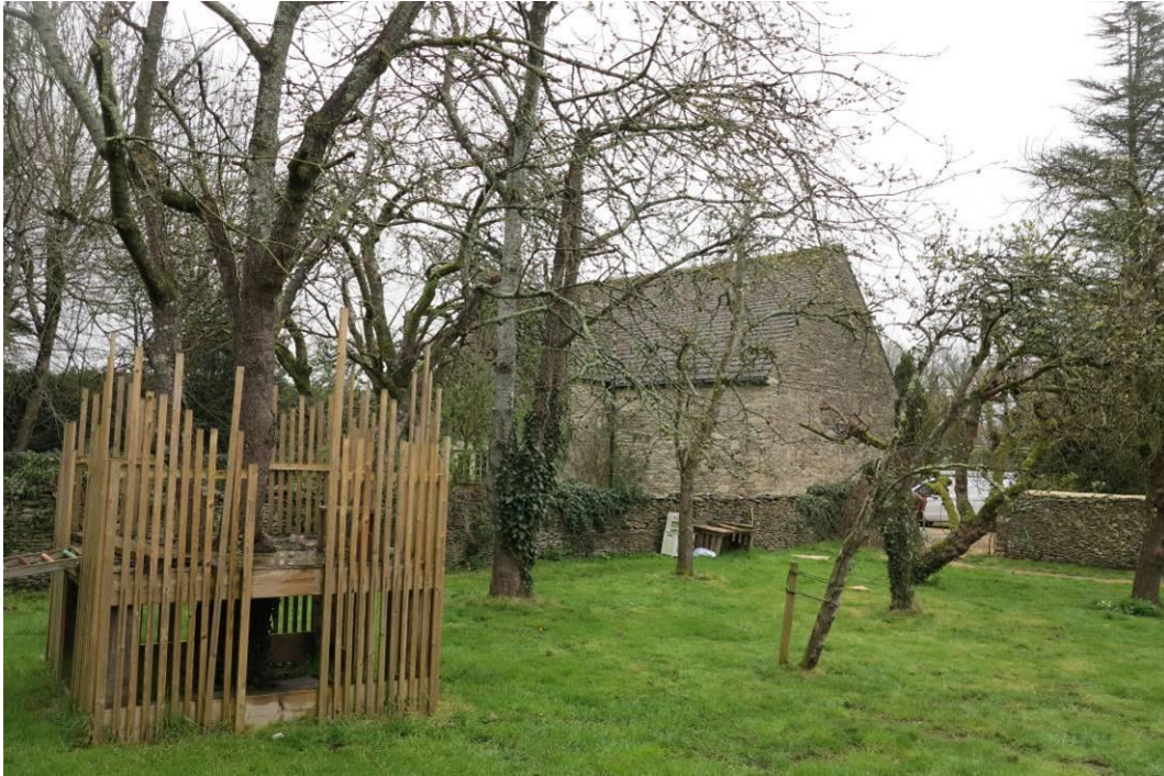
Plate 11. Listed barn seen across the orchard to the south
