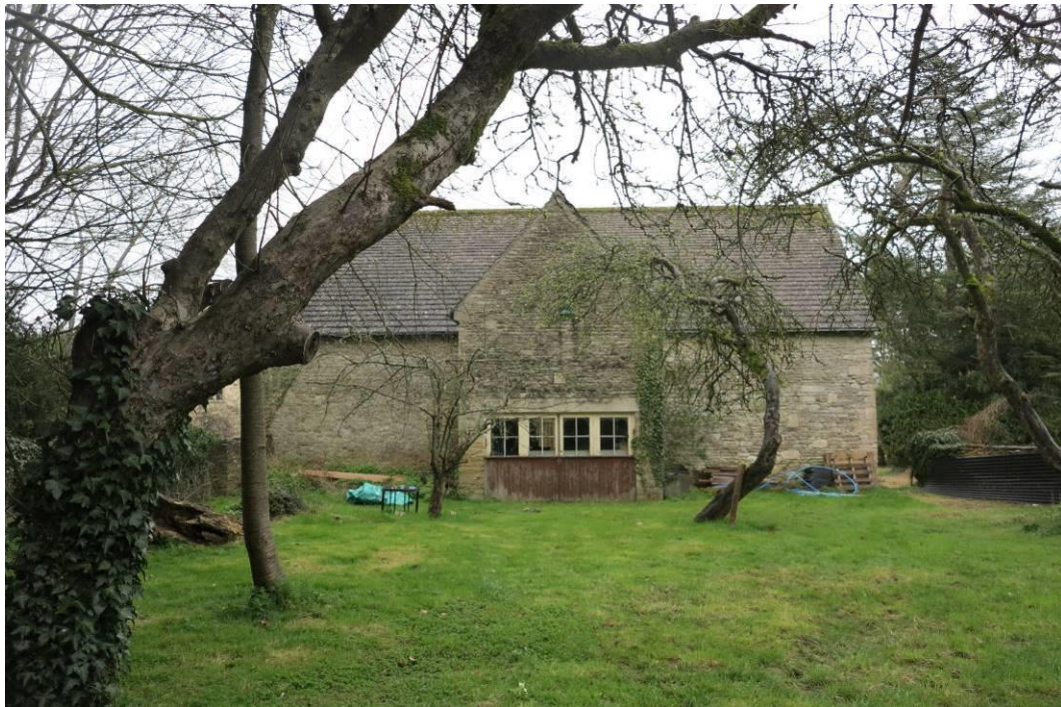
Plate 15. The south-western elevation of the barn, from the orchard located between the barn and the application site; note the visible elevation of the midstrey has been rebuilt
