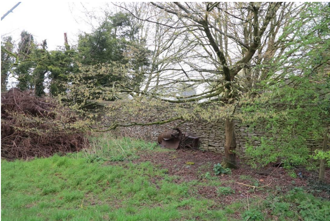
Plate 8. Drystone wall on the south-eastern site boundary
