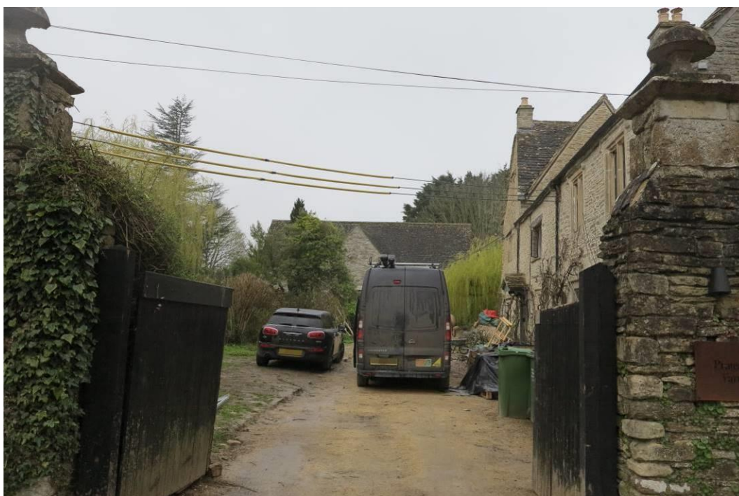
Plate 20. Praters Farmhouse and barn from the road access
