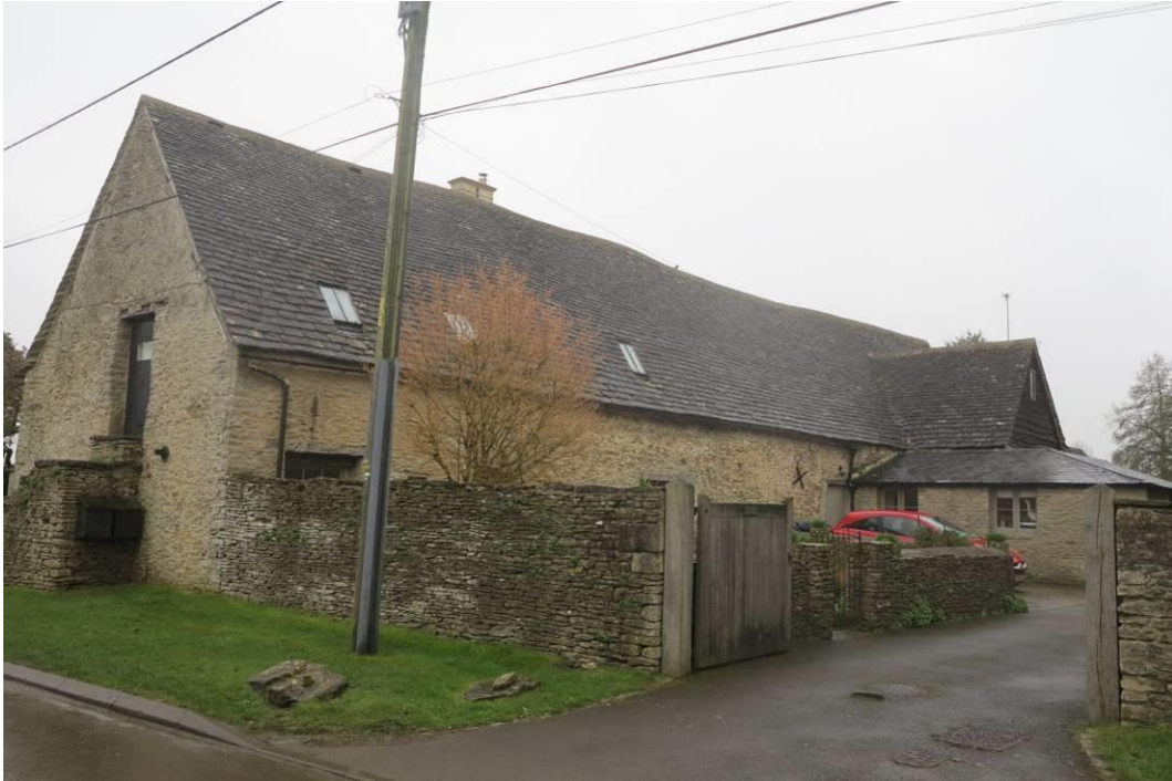
Plate 33. The listed outbuilding at Home Farm from the road
