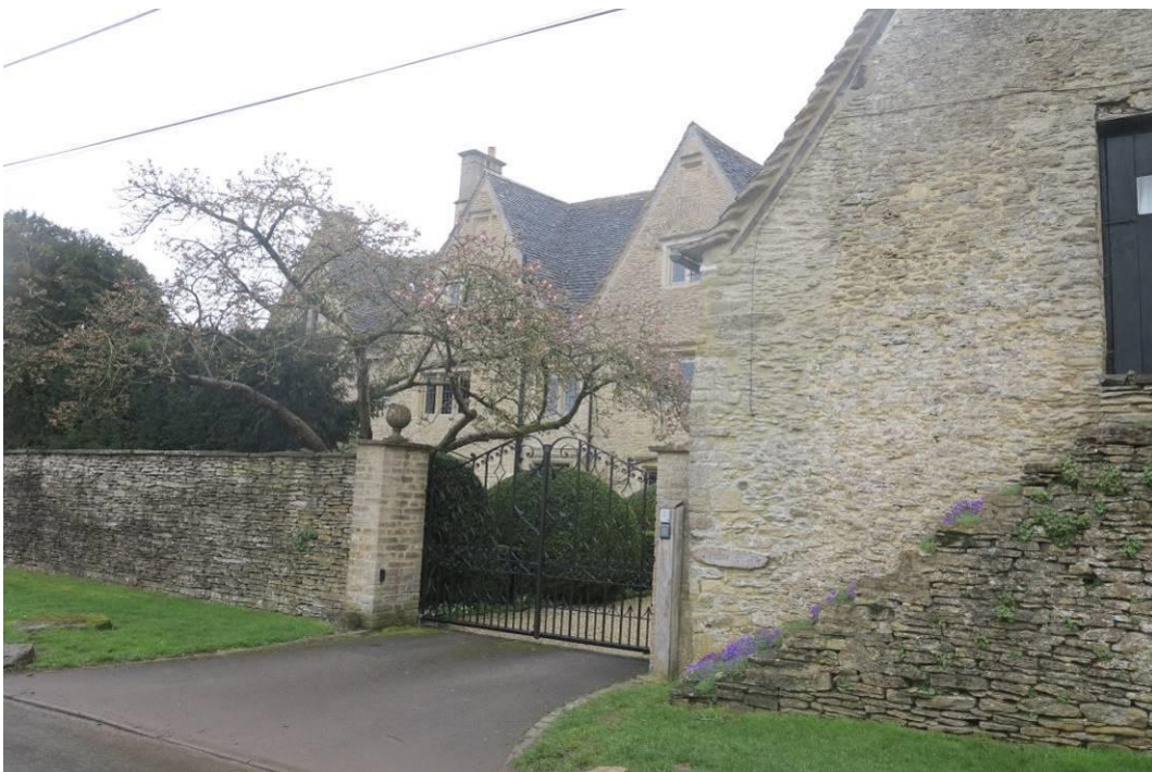
Plate 32. Home Farmhouse and its listed outbuilding from the road
