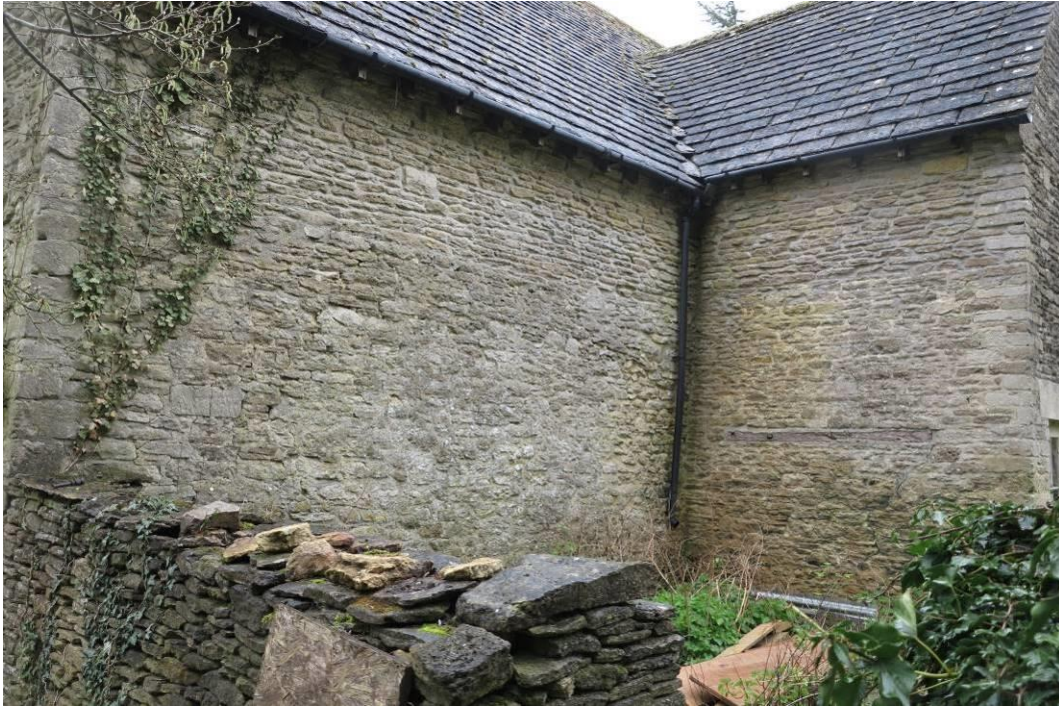
Plate 31. The south-western elevation of the barn; note the rebuilding of the upper element
