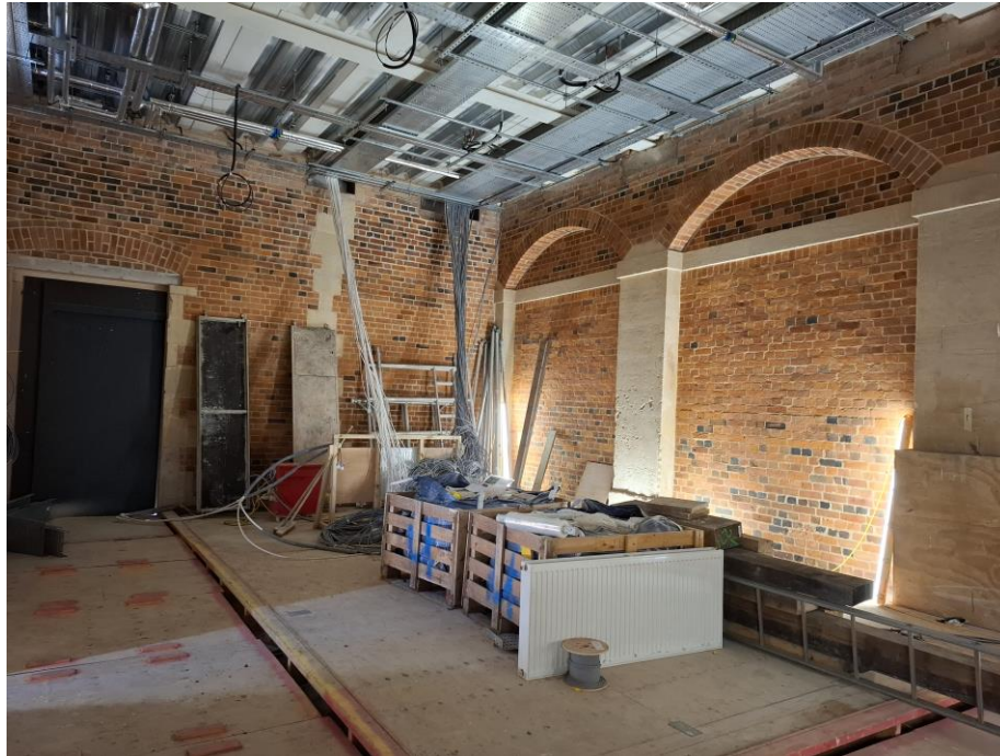
G22 (proposed Guest Bar) where the application of a breathable sealant to the exposed existing brickwork is deemed necessary.
