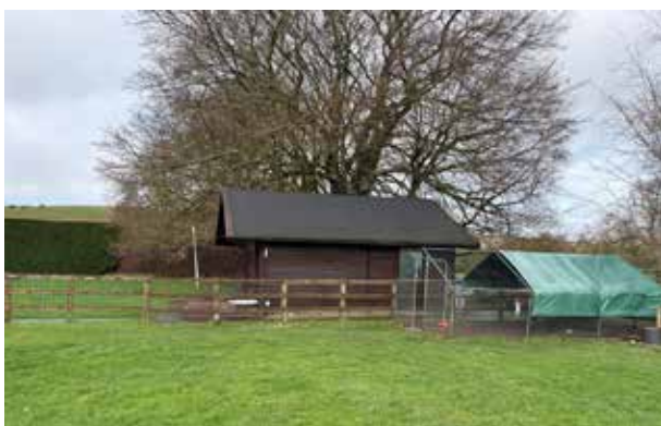
Fig 5 Existing Log Cabin - East Elevation
