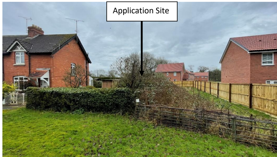
Figure 7: Application site looking north from access road
