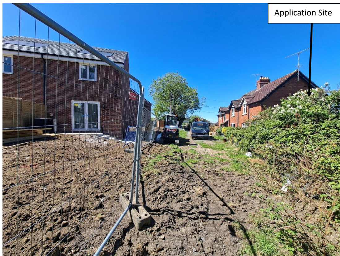
Figure 8: View of application site looking west towards the site (right) and development under construction
