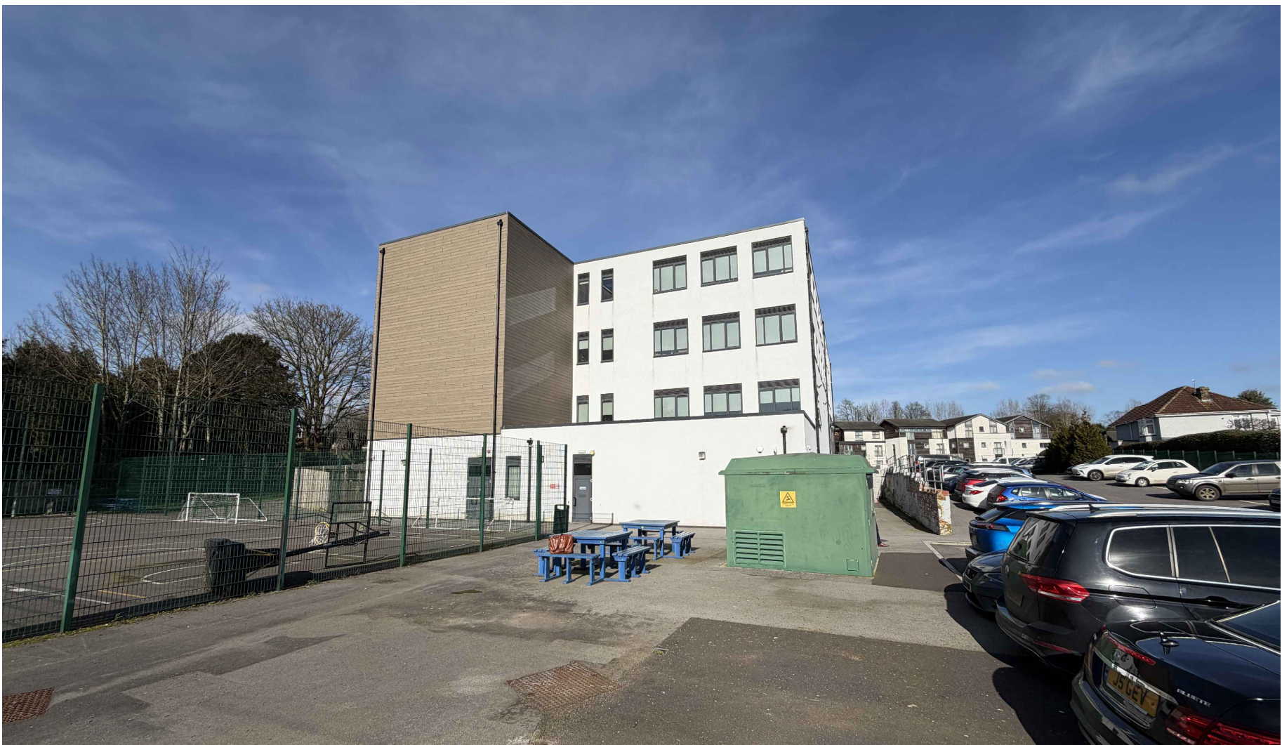
EXISTING BUILDING SOUTH ELEVATION
