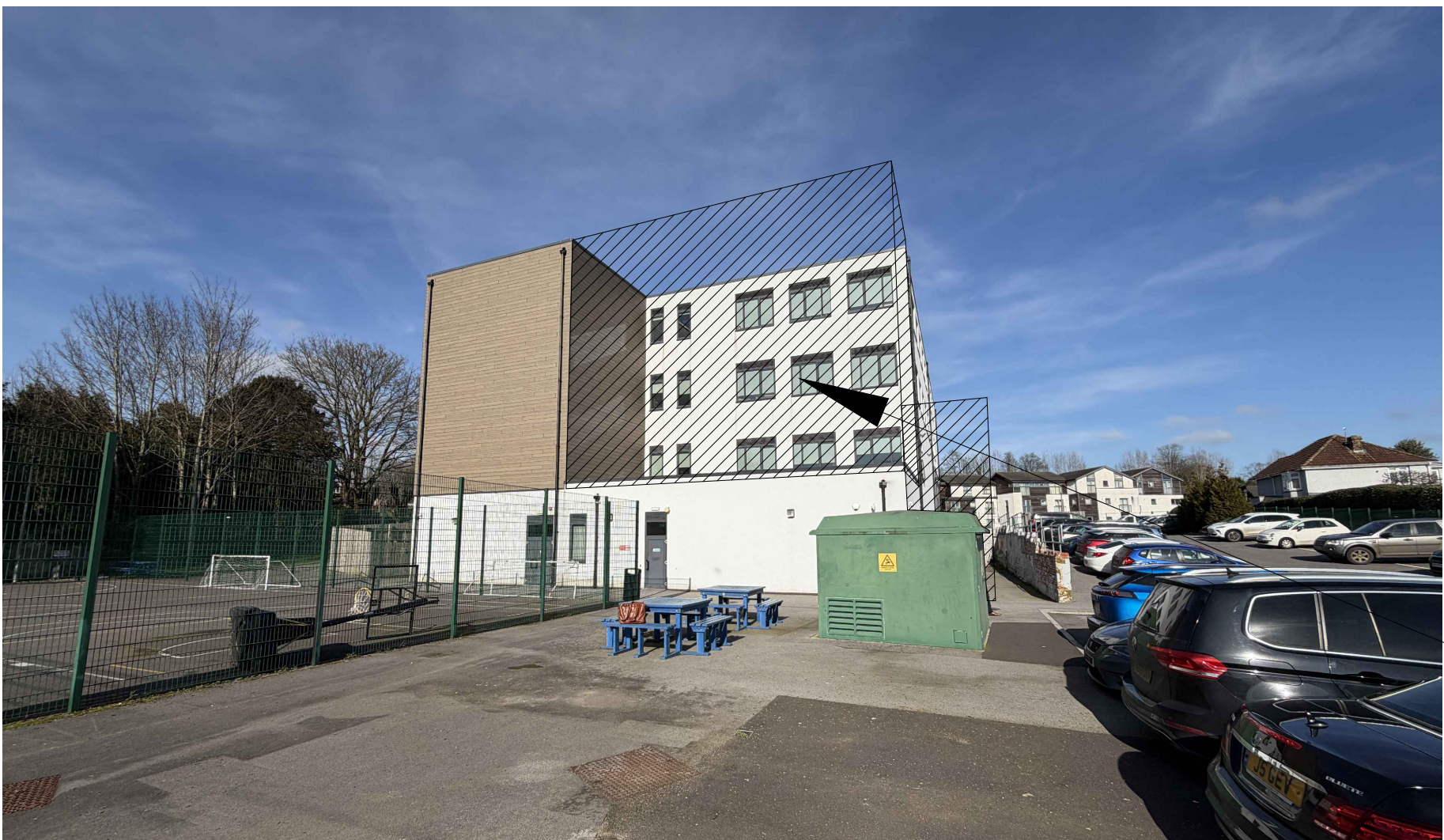
EXISTING BUILDING SOUTH ELEVATION
