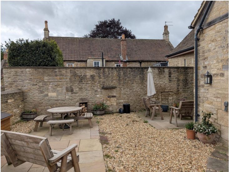
Photos 5, 6, & 7: East and west facing elevations of the Pope Barn (Barn 1), and view of shared boundary wall and private courtyard garden in the foreground
