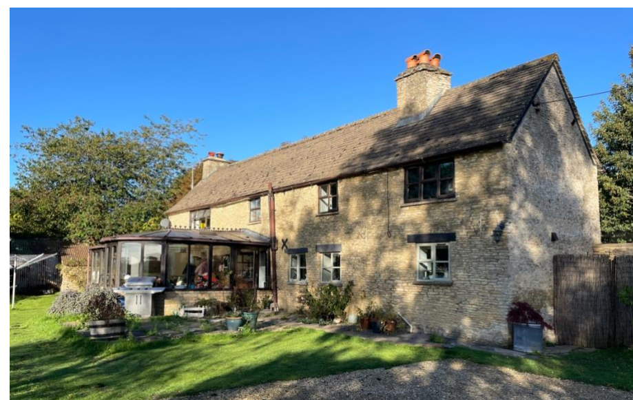
Fig 9 (Left) Knockdown Farm, former cottages north elevation, Fig 10 (right) former cottages south elevation
