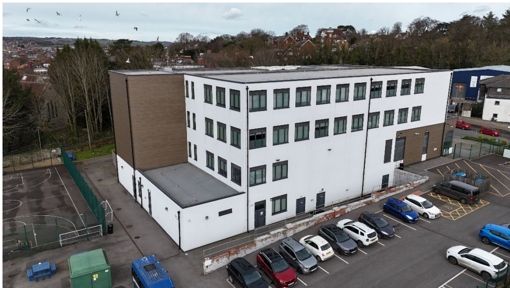
Photo 3 – East and South elevations of the existing building
