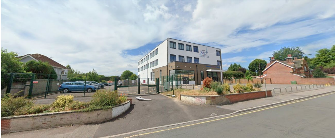
Photo 2 – Existing building. North elevation and site access from Tollgate Road
