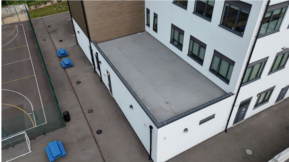
Photo 5 – Single storey, south east corner of existing building (location of proposed vertical extension)
