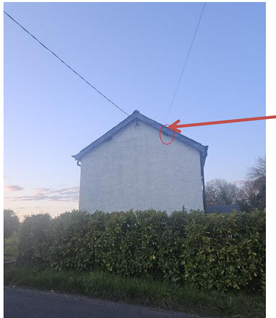
Figure 3: showing bat access/egress locations identified on the target building
