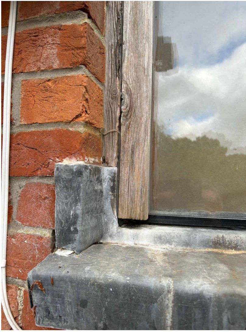
Existing cill detail - Proposed window to match
