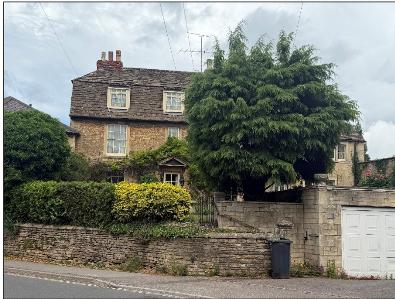
Image 13: Vine Cottage, front elevation from Marshfield Road
