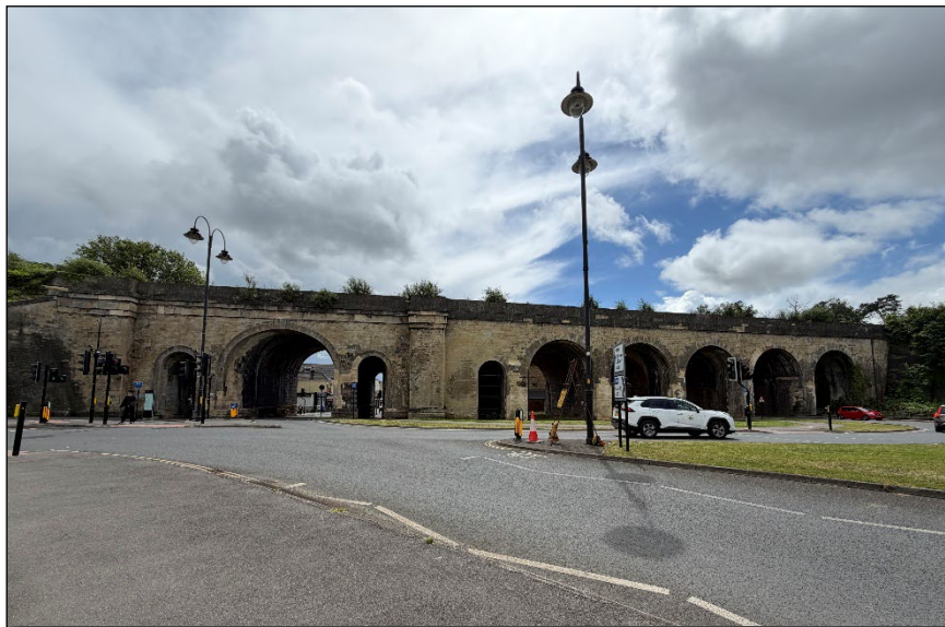
Image 17: Railway Viaduct, viewed from north
