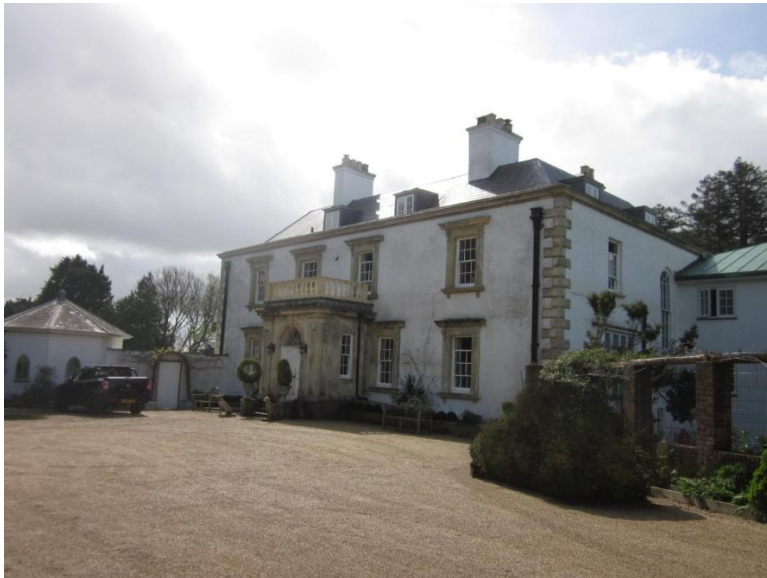
Main Entrance to Redlynch House
