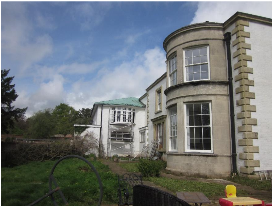
Rear of the property – South East corner with curved bay – present day
