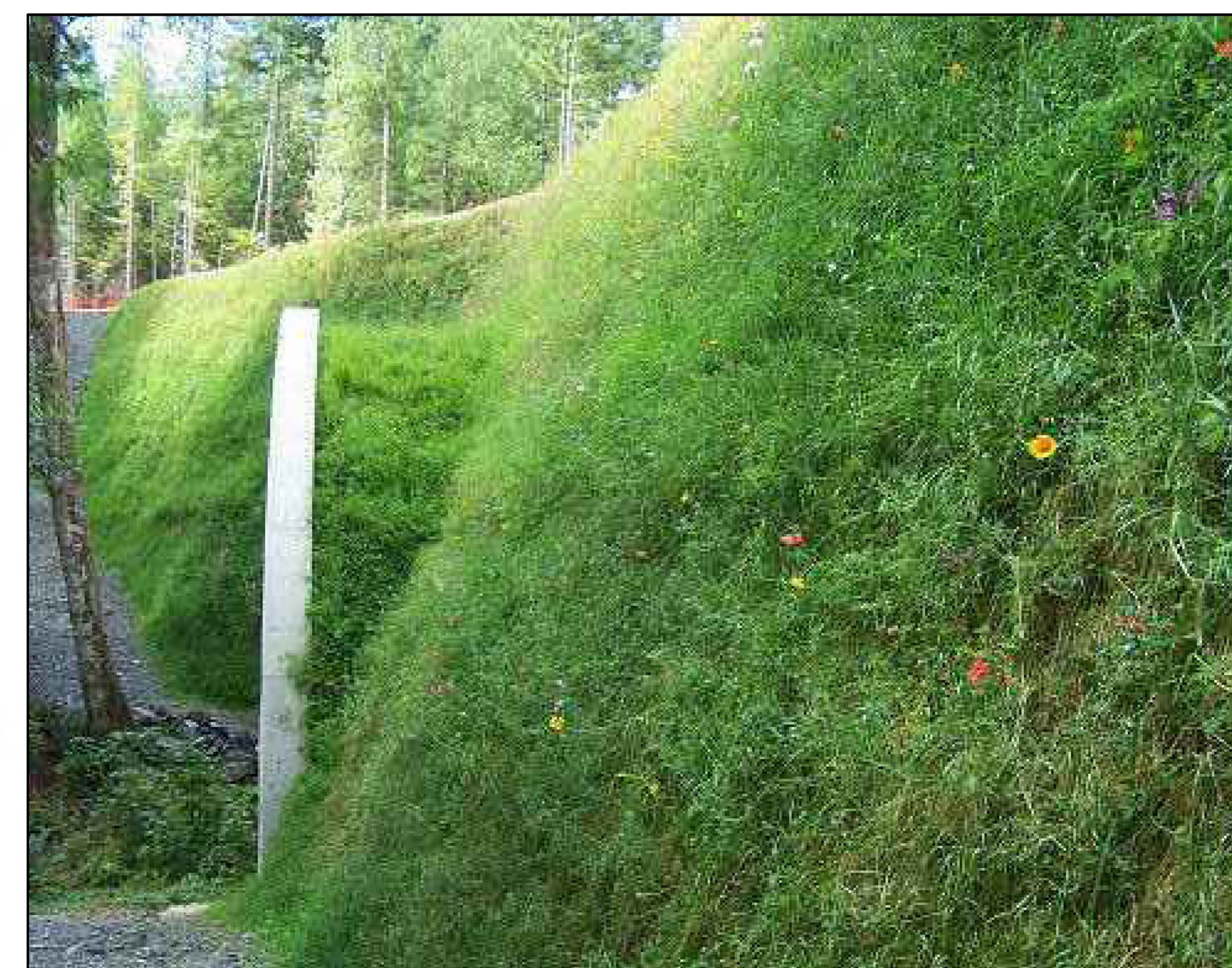
ROOTLOK VEGETATED WALL SYSTEM WITH CULVERT
