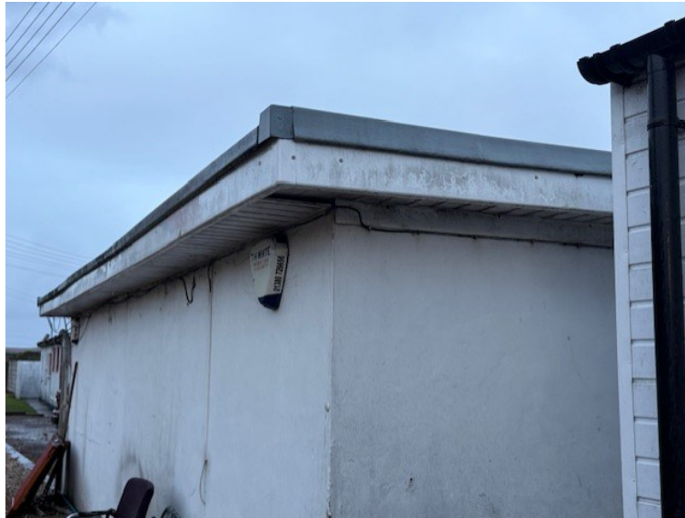
Figure 3: North western aspect of Building 2 with potential roosting features
