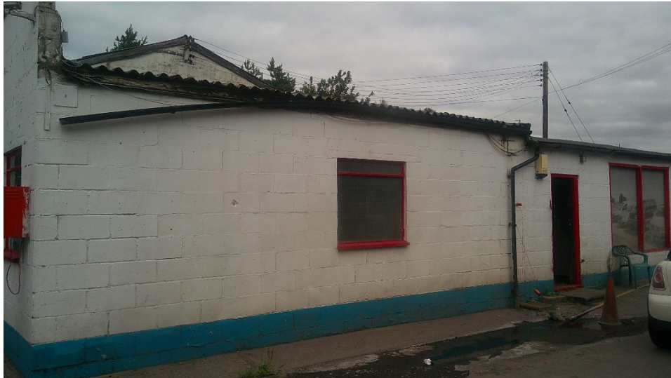
Northern Elevation of Building B4
