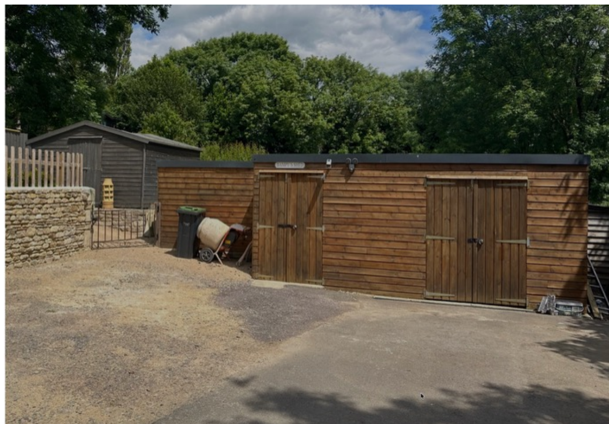
The Original ( now collapsed) building to be Replaced
