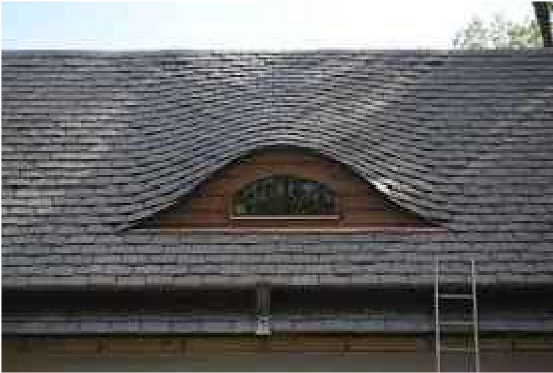
EXAMPLE PHOTOGRAPH OF EYEBROW DORMER FINISHED IN SLATE Scale - N.T.S
