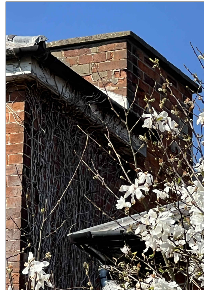
Existing chimney to reinstated (Northeast)
