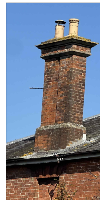
Existing chimney (Southwest)
