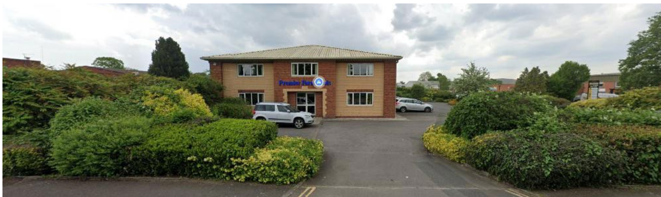
5. View of Premier Form Tools, 1 Lancaster Road (adjacent to site West elevation)
