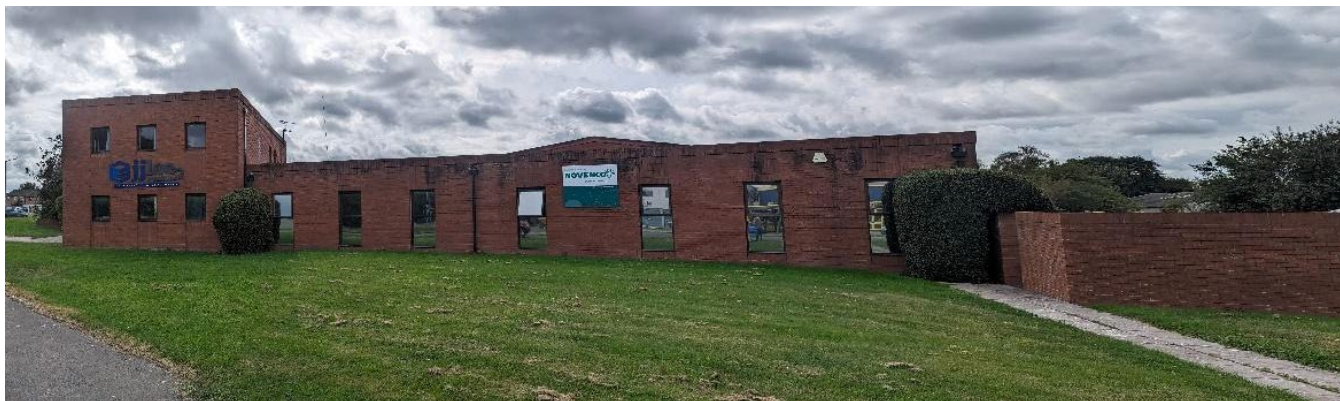
1. View of the Existing building North elevation
