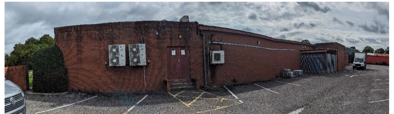
2. View of the Existing building West elevation
