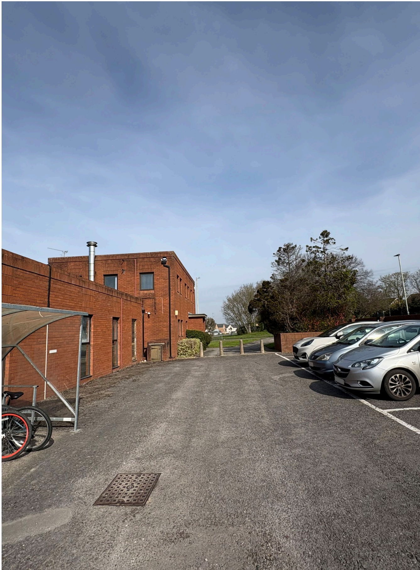
View of the Existing building East elevation
