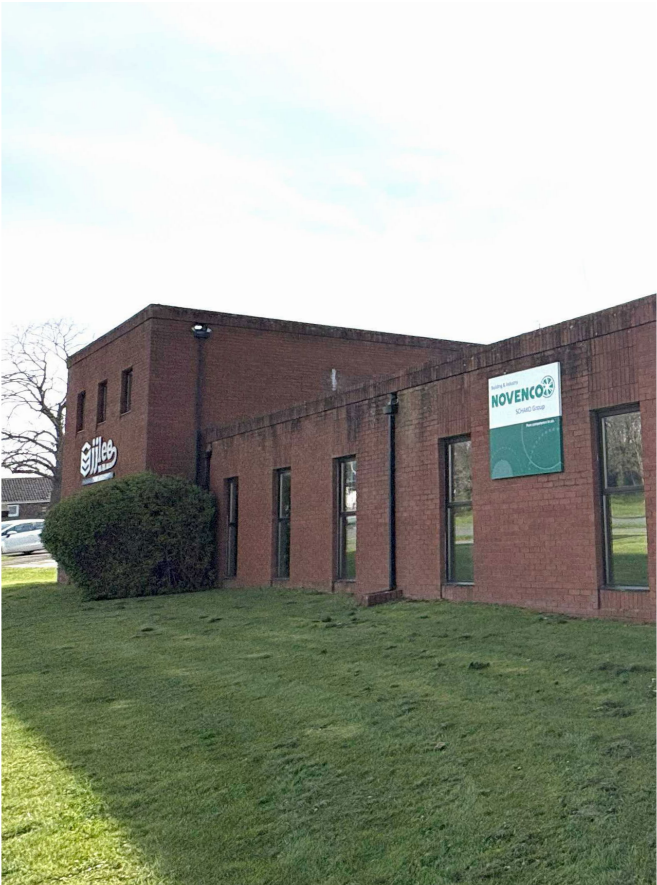
View of the Existing building North elevation
