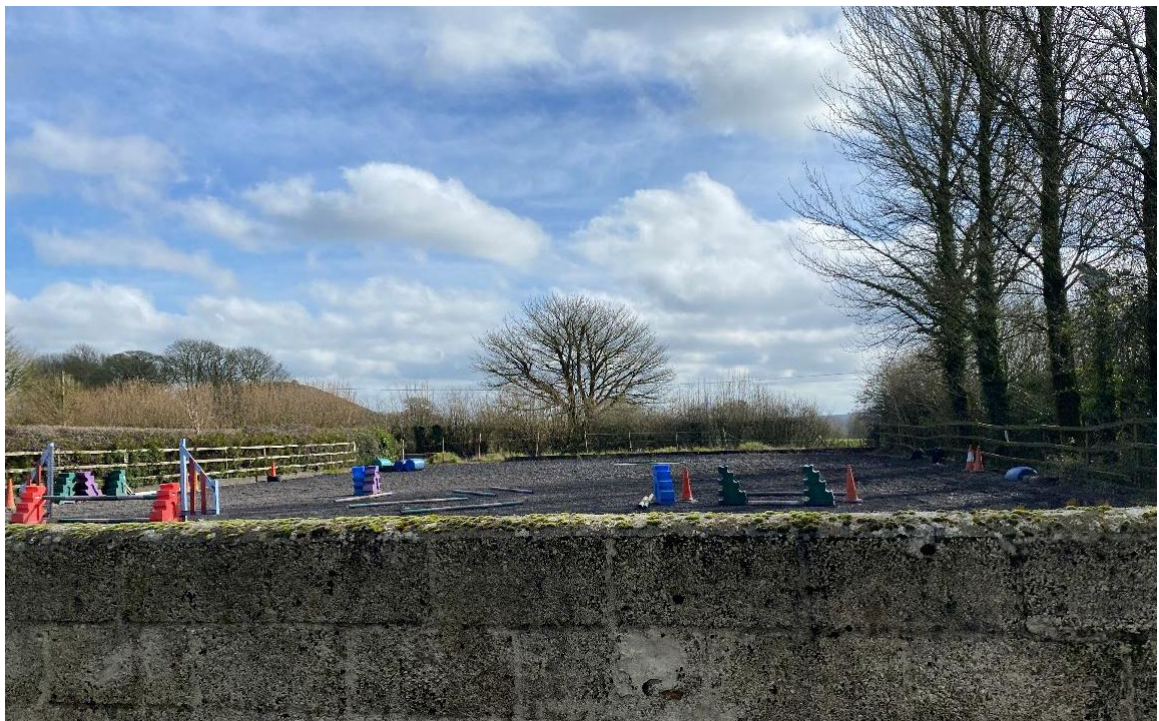
Figure 6 - Modern menage and concrete block wall to be removed and returned to grassland
