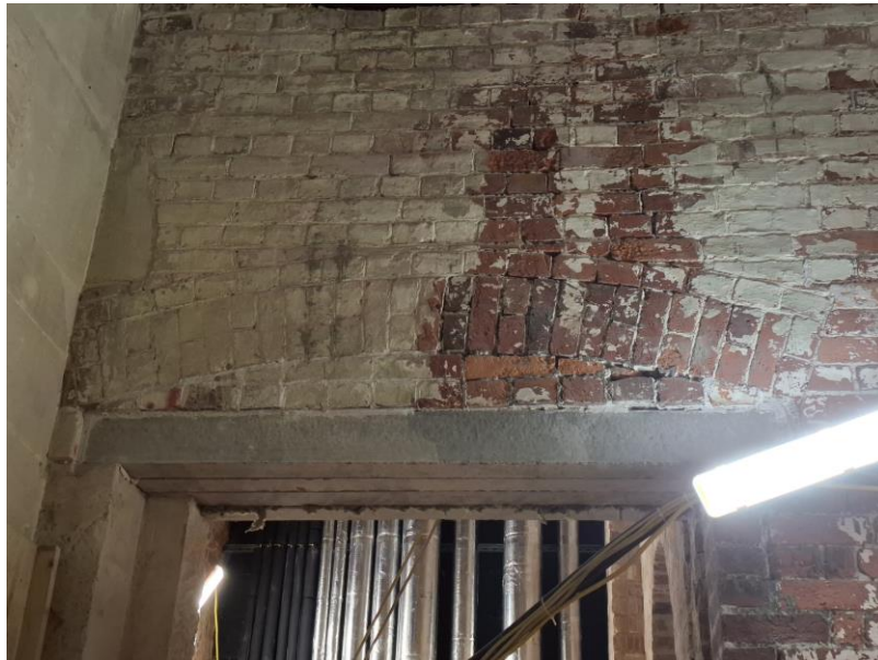
Brickwork above DG19
