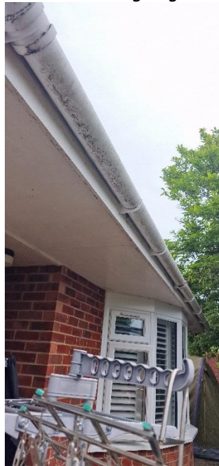
Picture 6: The soffits
