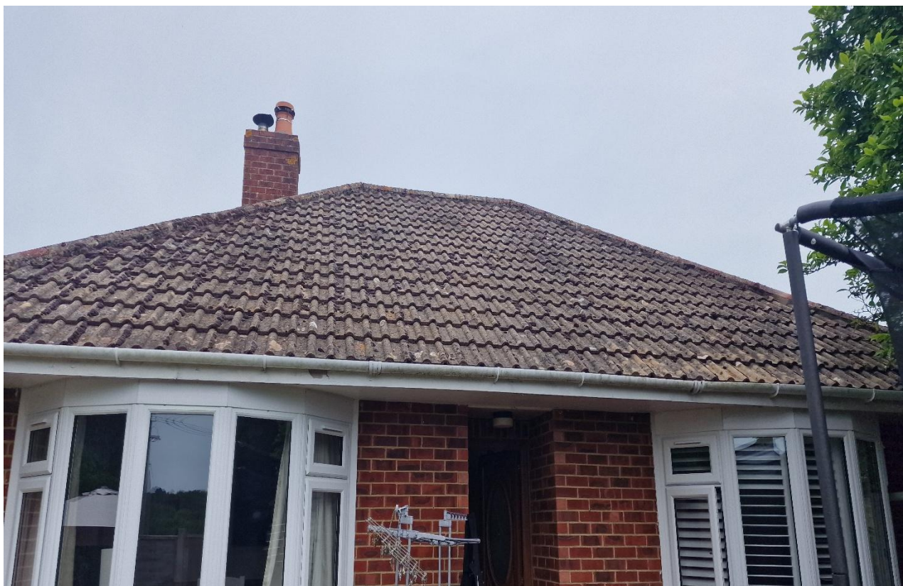
Picture 3: The side elevation of the property
