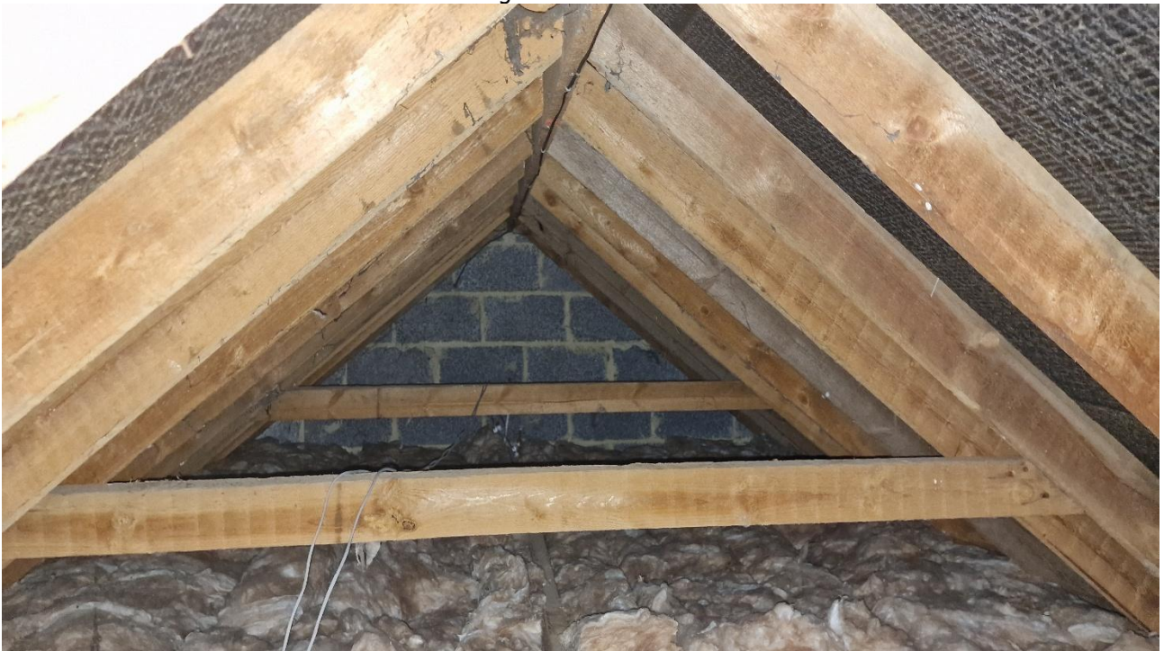
Picture 10: Showing the internal structure of the roof
