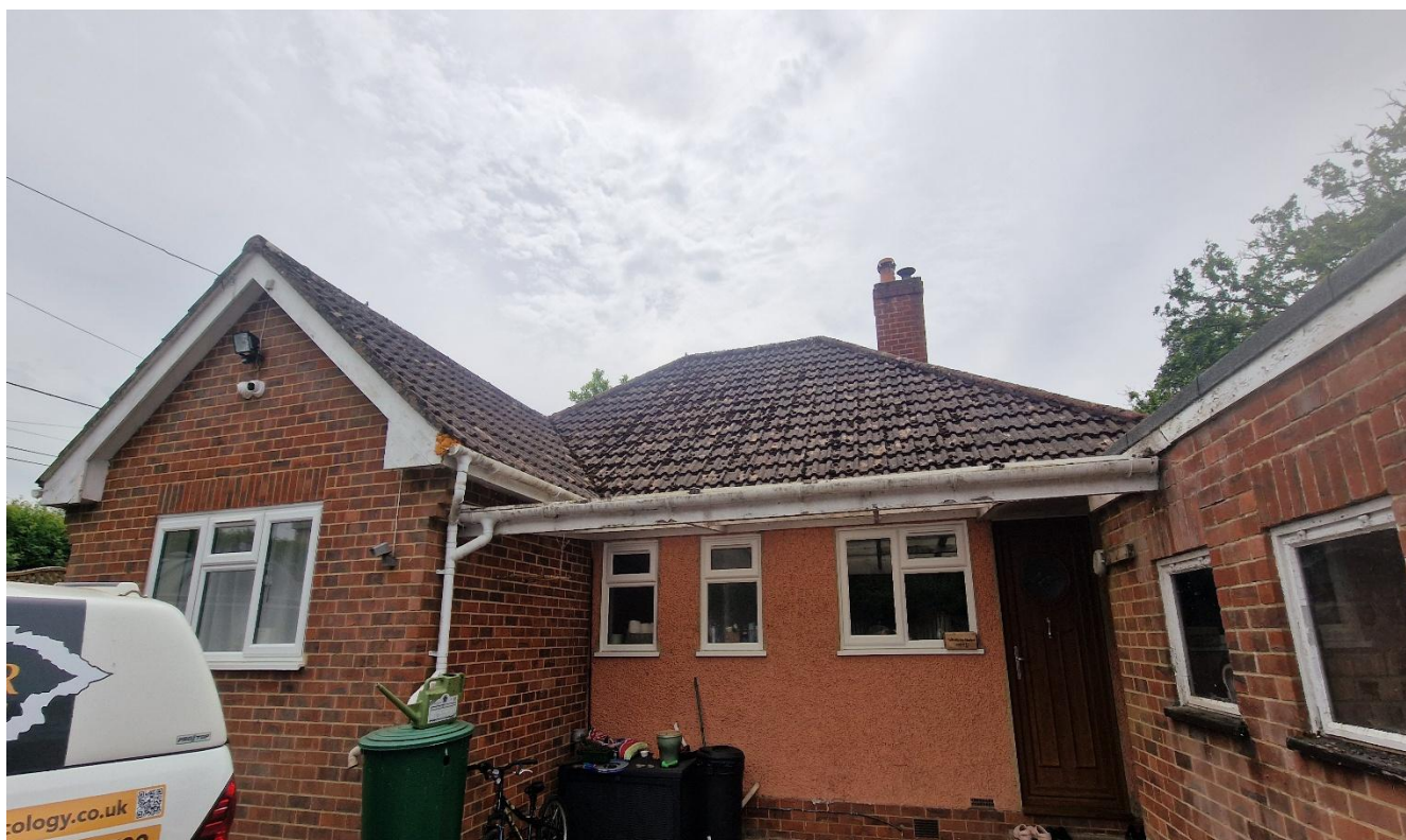
Picture 4: The side elevation of the property
