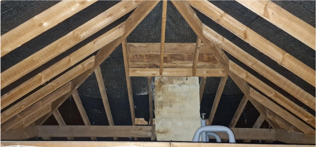
Picture 9: Showing the internal structure of the roof
