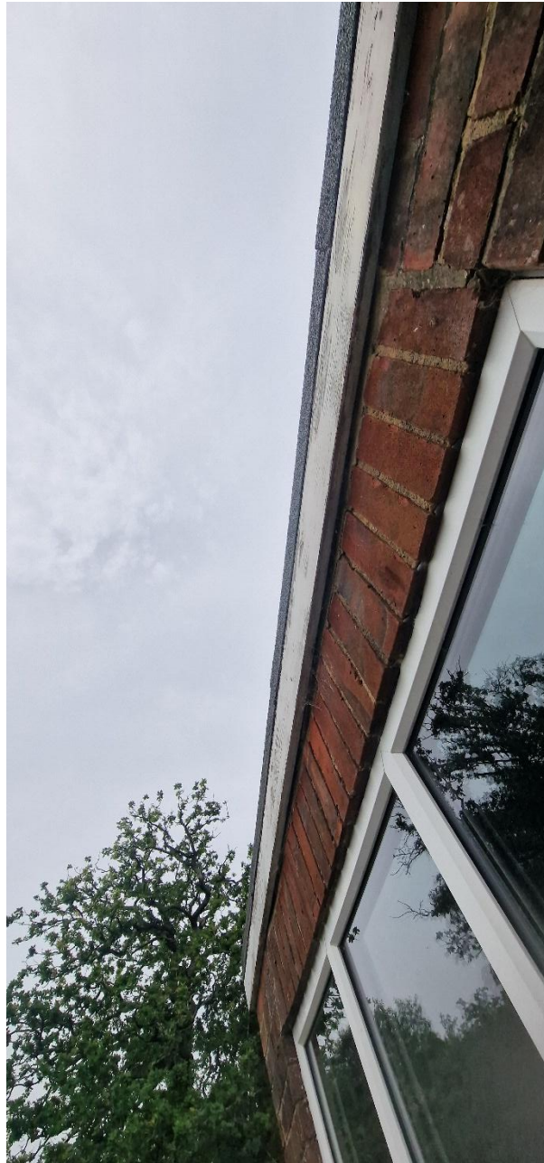
Picture 8: The garage barge board
