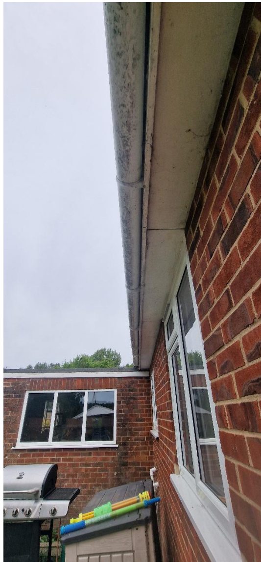
Picture 7: Showing the soffits
