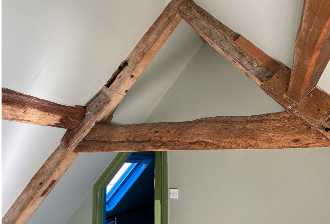
Figure 27: Exposed roof truss showing empty mortices from the altered form.
