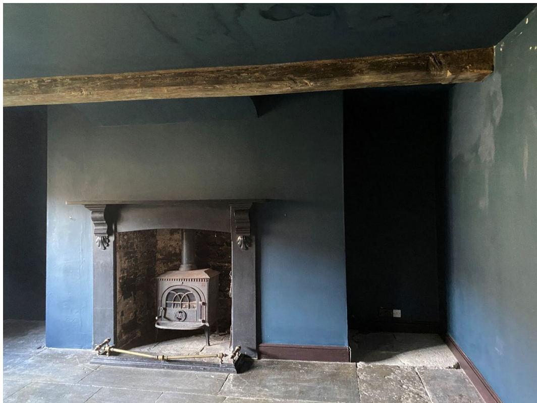
Figure 24: Robust slate fire place surround in ground floor space, likely authentic and in situ.
