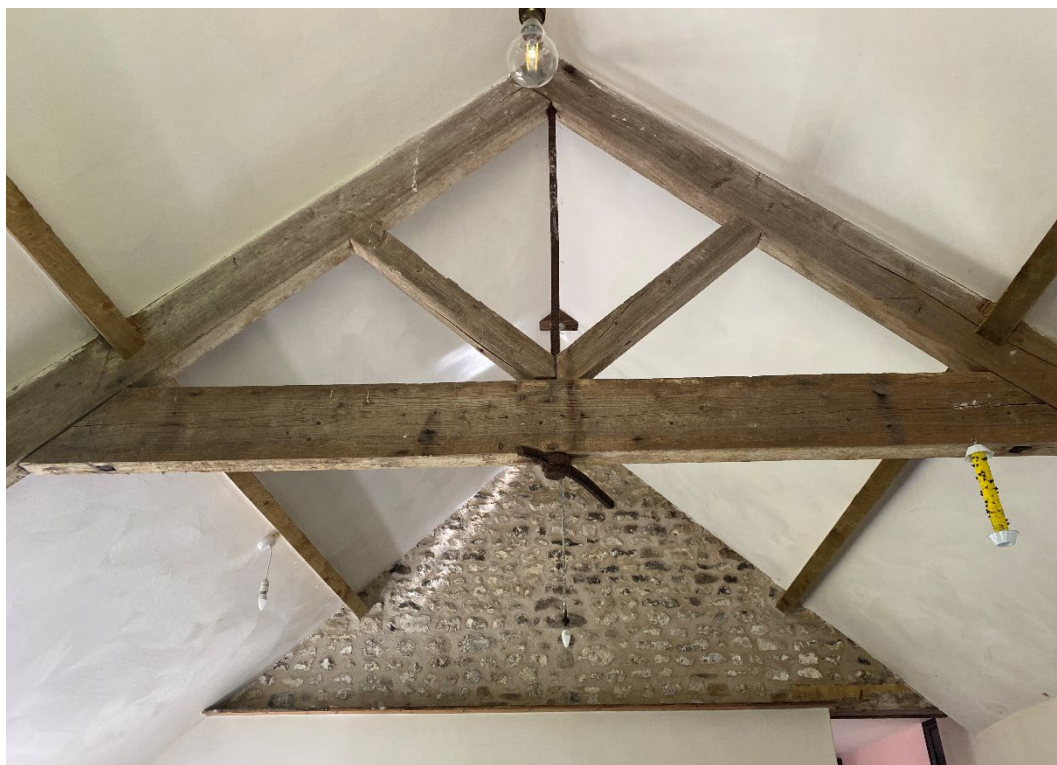
Figure 19: Interior with exposed roof truss in the lower portion.
