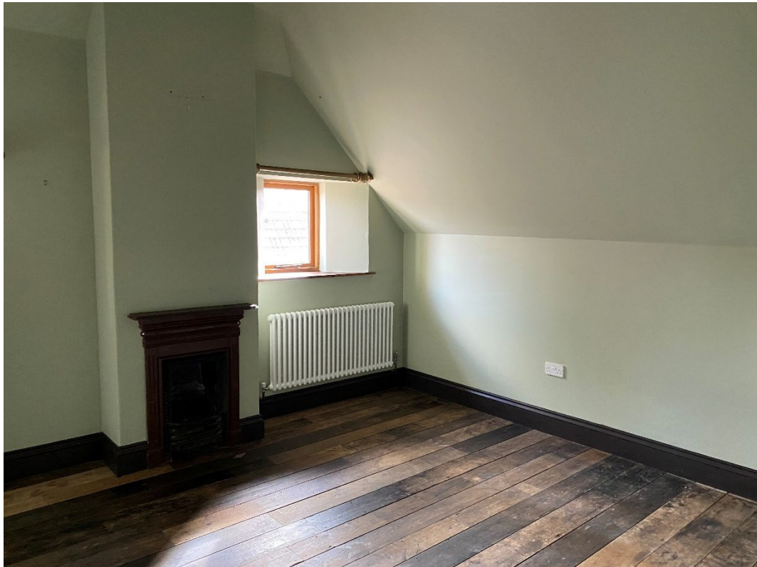
Figure 21: Typical quality of the first floor rooms.
