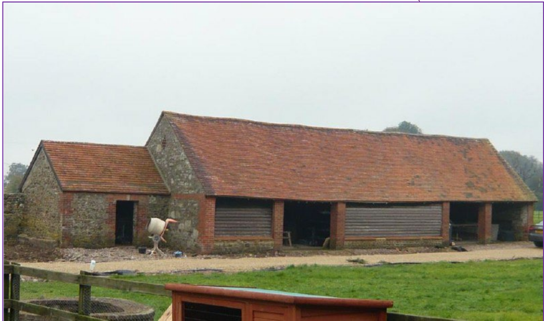
Figure 11: The southern range in 2014 prior to conversion (Elaine Milton Heritage and Planning, figure 26, p.19)
