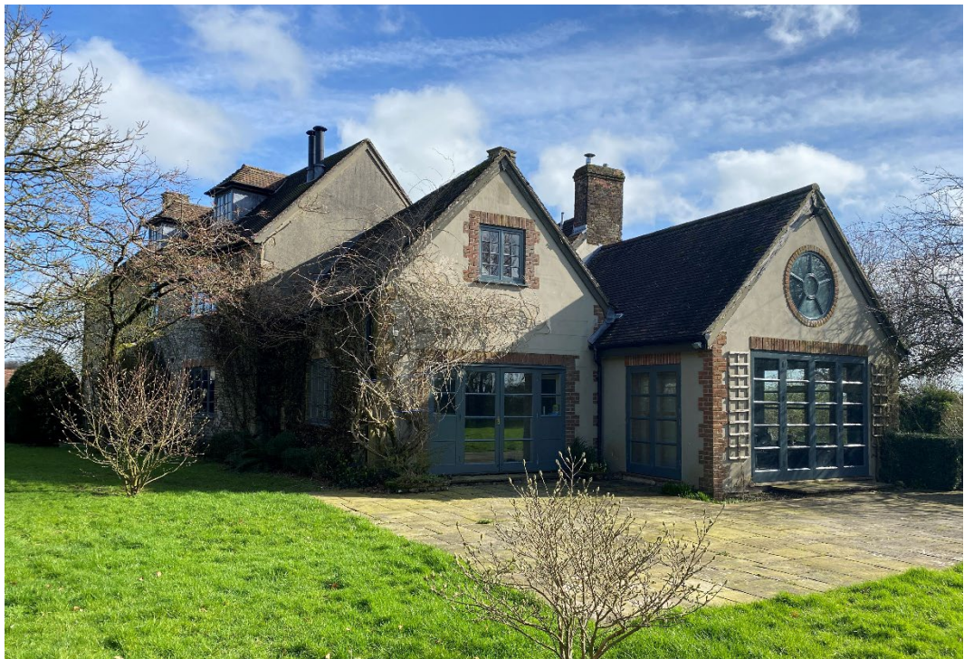
Figure 23: Recent extensions added to the house's western elevation.
