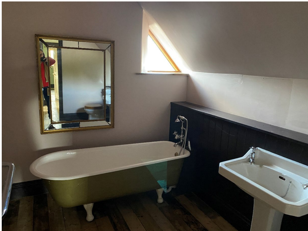
Figure 37: The existing bathroom to be renewed and adjusted. Note comparative darkness which will be alleviated through two small conservation roof lights.
