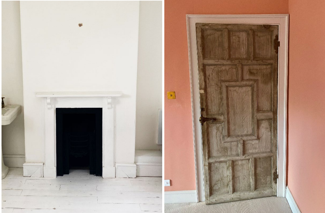
Figure 25-26: Small iron grate and simple surround in western portion, ornate imported door in main first floor space.
