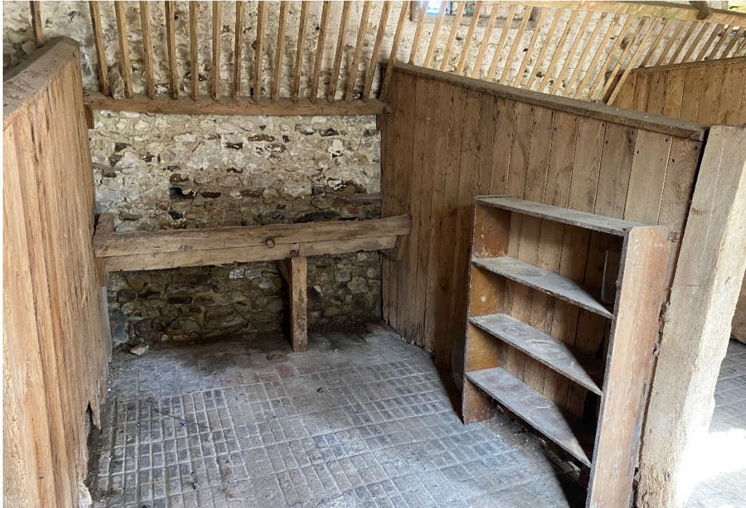
Figure 29: Simple but functional stall dividers, trough with tether ring, hay rack and moulded block floors and ventilation grilles.
