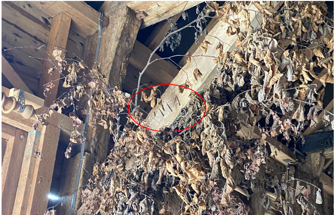
Figure 5: Carved date '1774' on a brace adjacent to the south western threshing door, the '7's are carved backwards.
