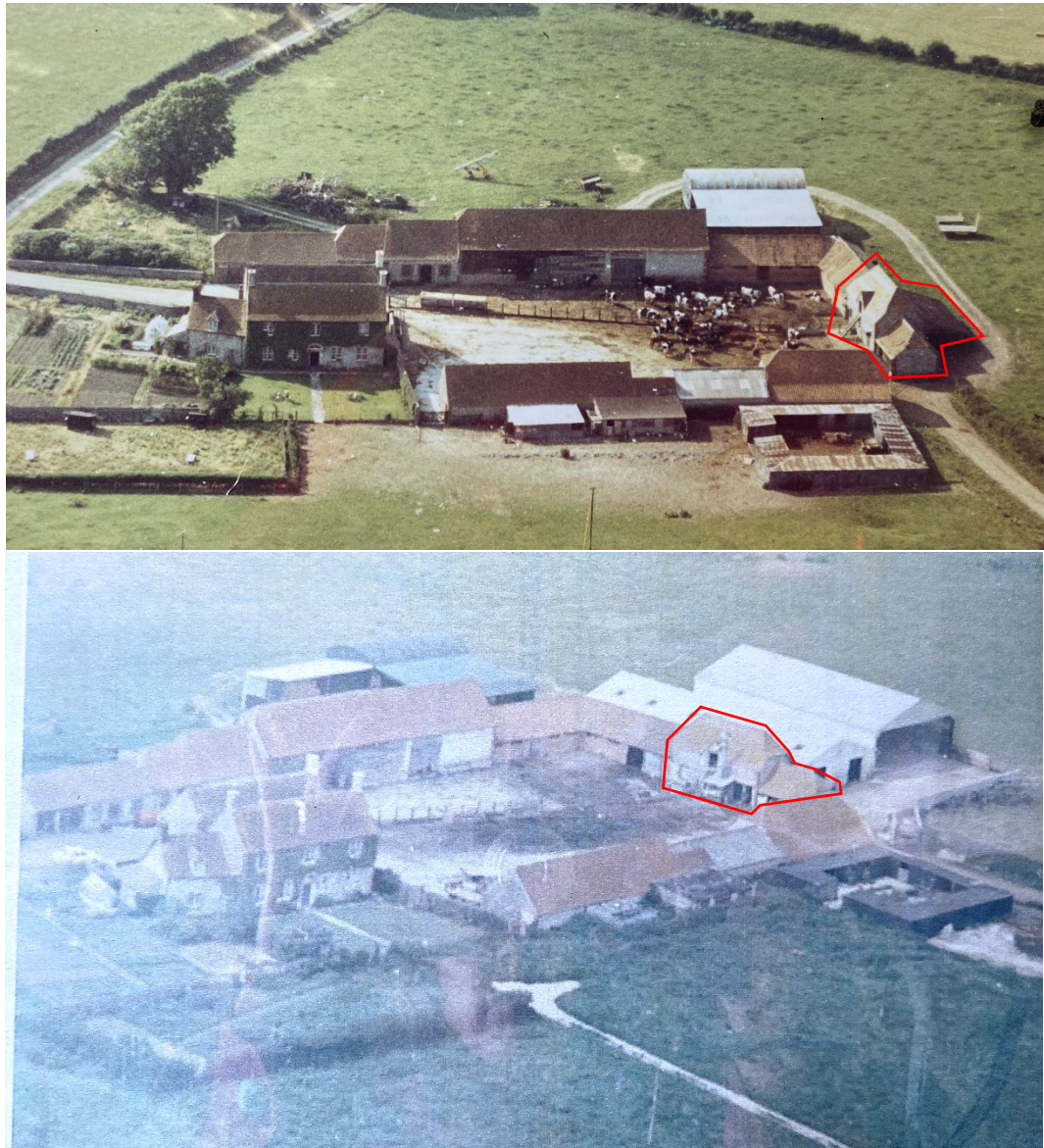
Figure 13: 1980s photographs, when the farm was still in active use. Note cows in yard, additional structures to the south and north, and then to the north east, firm access from the north east and north west. A path reinstated to the southern front in the lower one, no longer present.
