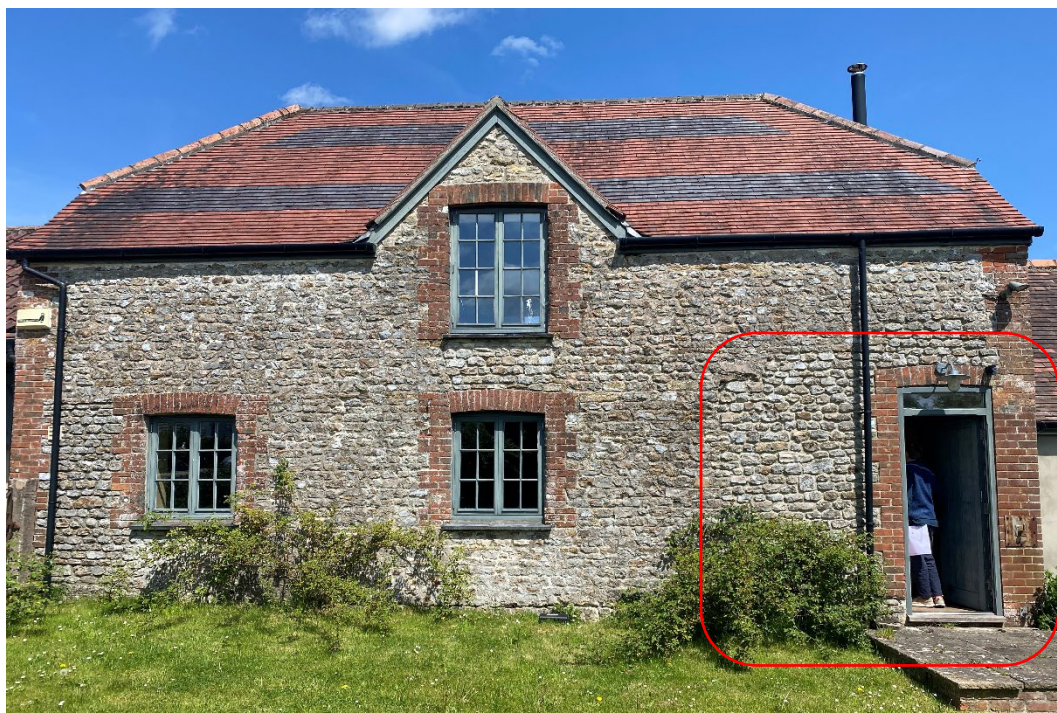
Figure 17: Front elevation note slightly different stone character in area of former opening.
