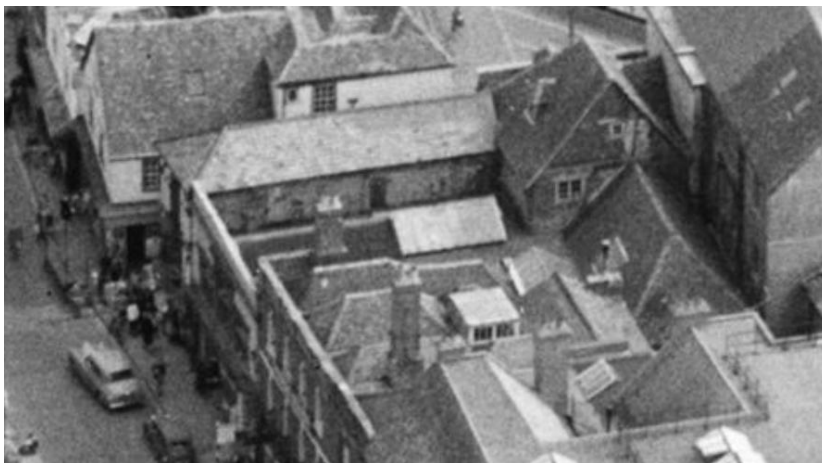
1953 A large presumably glazed section forms the rear/south part of the roof, surrounded by a variety of flat sections.
