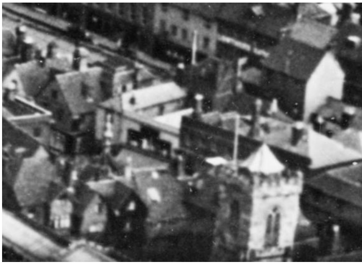
1924. NB White area of roof behind parapet in centre of image. This seems most likely to be a shallow slate roof.
