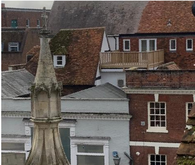
2026 (applicant) All of the roof has a felt covering. More photos on file.
