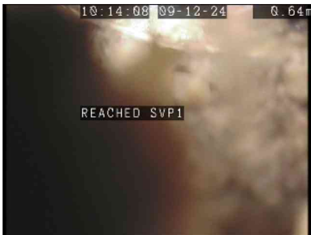
SVP1X_b13e51bf-72bd-45b3-9aee-96f57d9fdb9a_20241211_124557_556.jpg, 00:00:31, 0.64 m Finish survey, Reached base of SVP1
