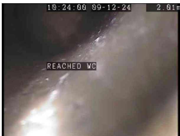
WCX_0d71509d-2fa0-4a63-bc4a-5b50825fb1ef_20241211_125325_655.jpg, 00:00:28, 2.01 m Finish survey, Reached base of WC
