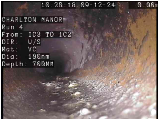
IC2X_0ca80de5-28c6-42d6-92c6-dc64ecbcec74_20241211_125117_033.jpg, 00:00:00, 0.00 m Start of survey
