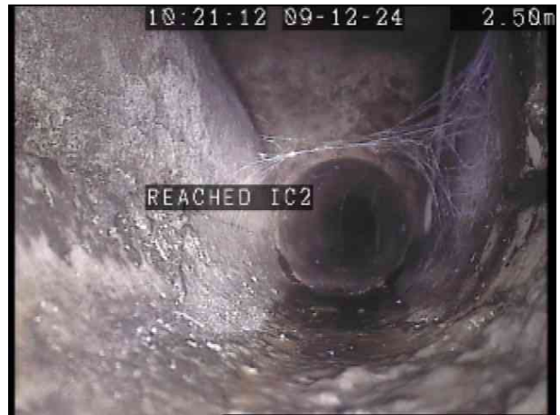
IC2X_f72b5f12-76c6-4d12-9ad0-5988b03c946f_20241211_125213_000.jpg, 00:00:38, 2.50 m Finish survey, Reached IC2
