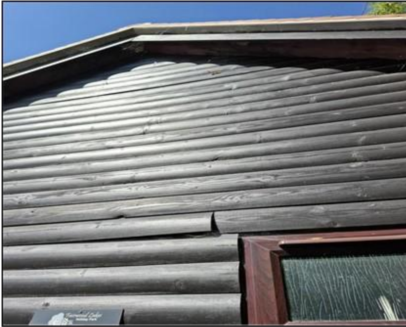
Photograph 3 showing cladding on shower block
