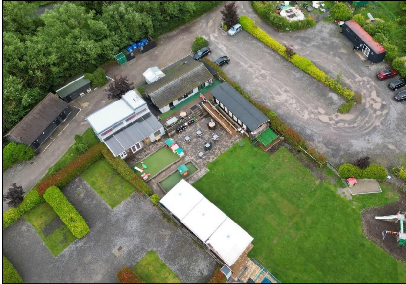
Photograph 2 showing café building, with soft play zone and railway carriage adjacent
