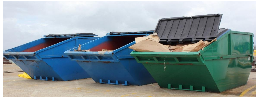
Segregated waste category skips within designated site zone
