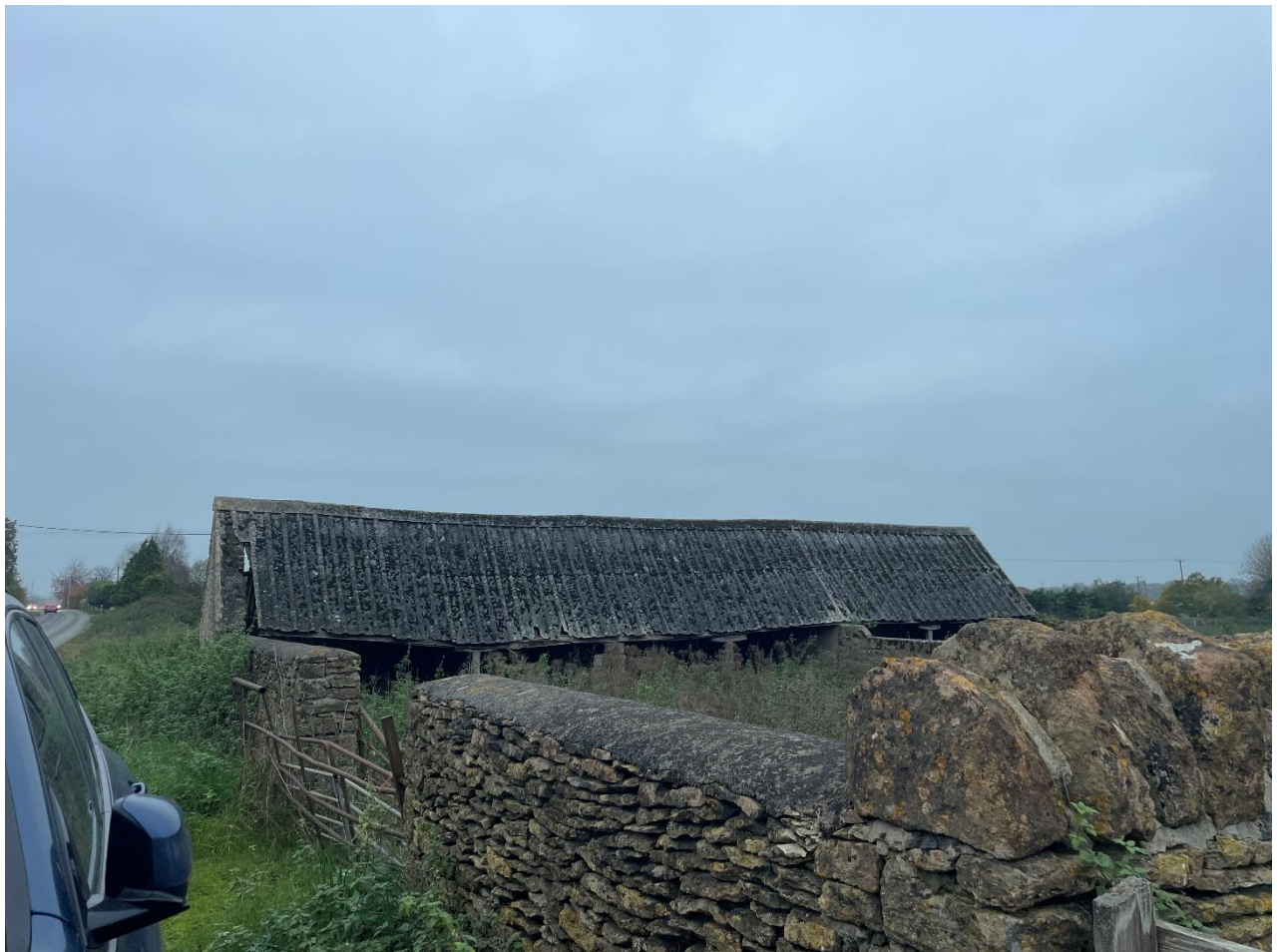
Figure 4.7 The Shelter Shed to the east of the B4643
