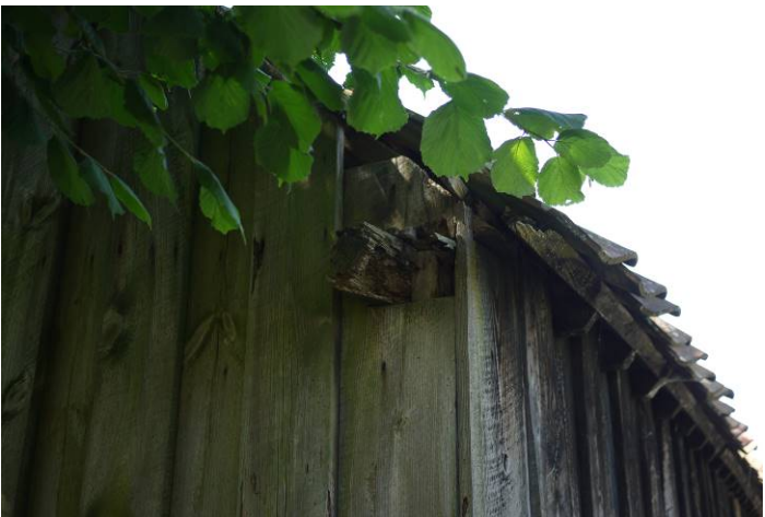
Photo 7. The rotated wall between trusses 1 and 3
