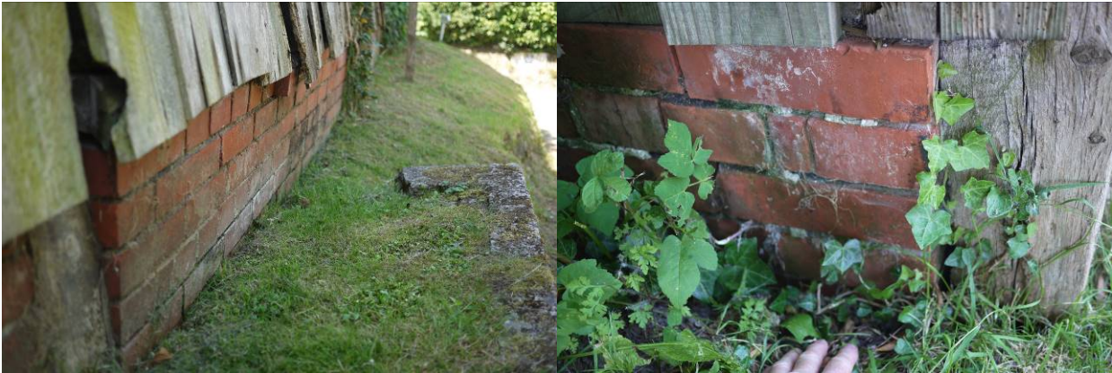
Photo 7. The rotated wall between trusses 1 and 3
