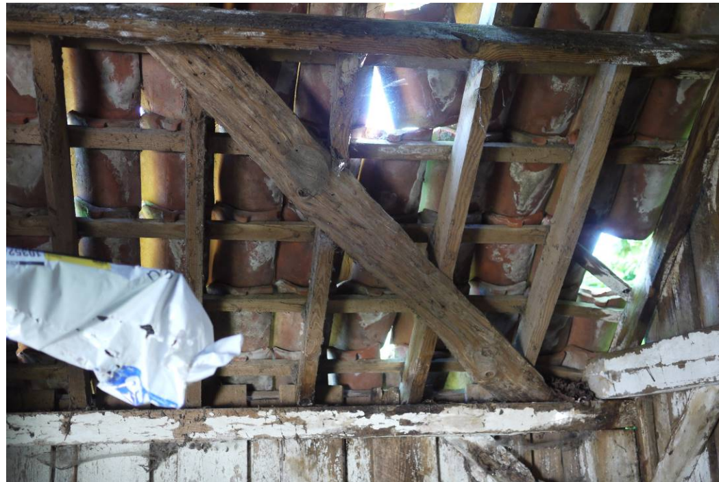
Photo 12 – showing the poor quality and rot in the purlins which are to be replaced.
