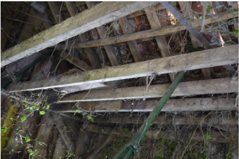
Photo 6. The underside of the roof adjacent Truss 1
