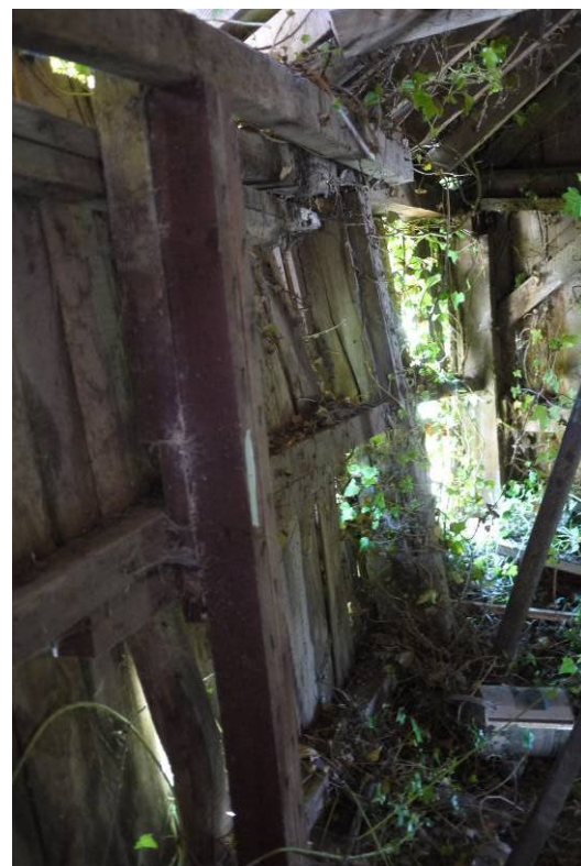
Photo 12 – showing the poor quality and rot in the purlins which are to be replaced.
