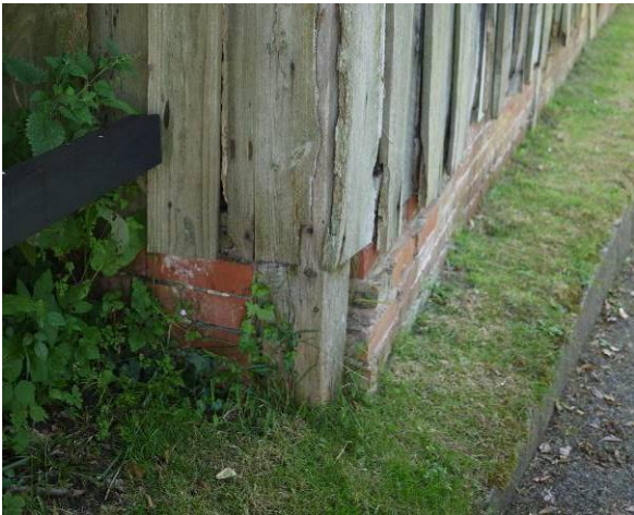
Photo 2. North east corner showing earth-bound principal
