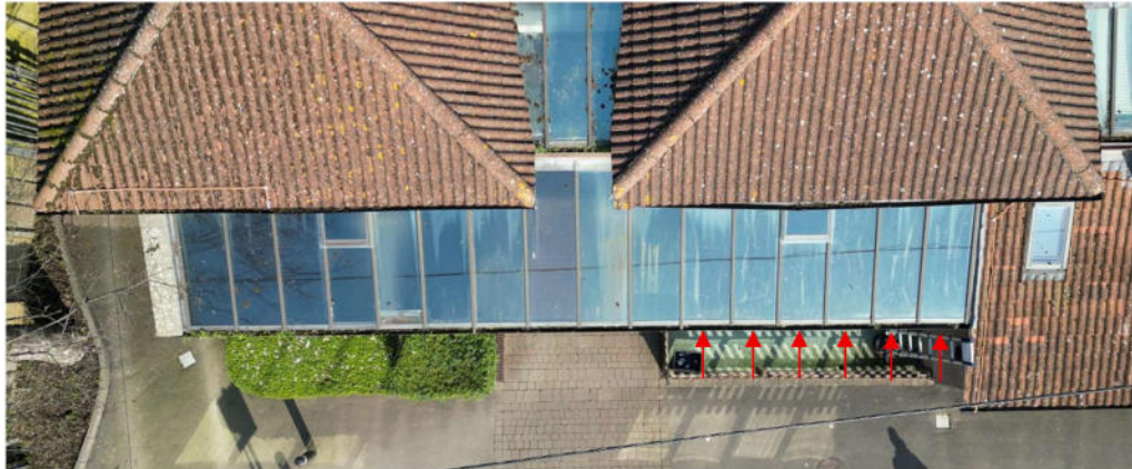
Image 3: Aerial Image of Lean-To Roof.
