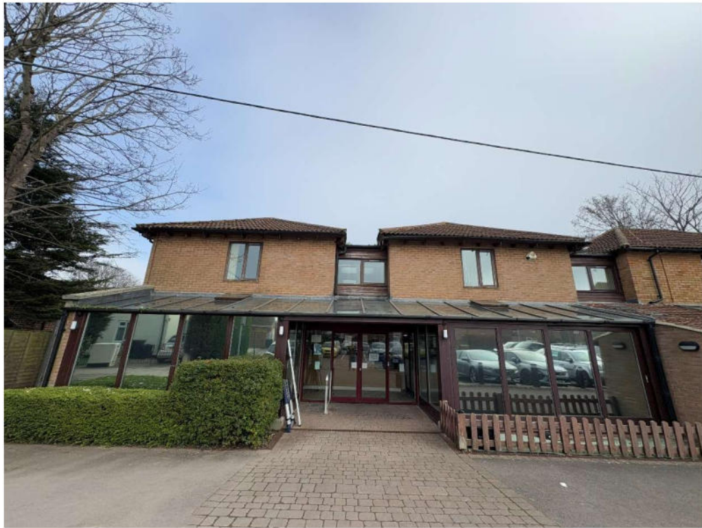
Image 1: Existing Lean-to Structure (South Elevation).
