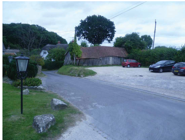
Fig. 1 - View of the barn from the south
