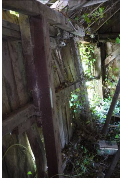
Fig. 9. The internal south west corner showing props.
