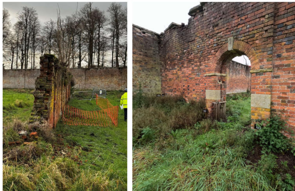
Figure 10 - Historic photographs of Spine Wall, Opening 3 on RHS
