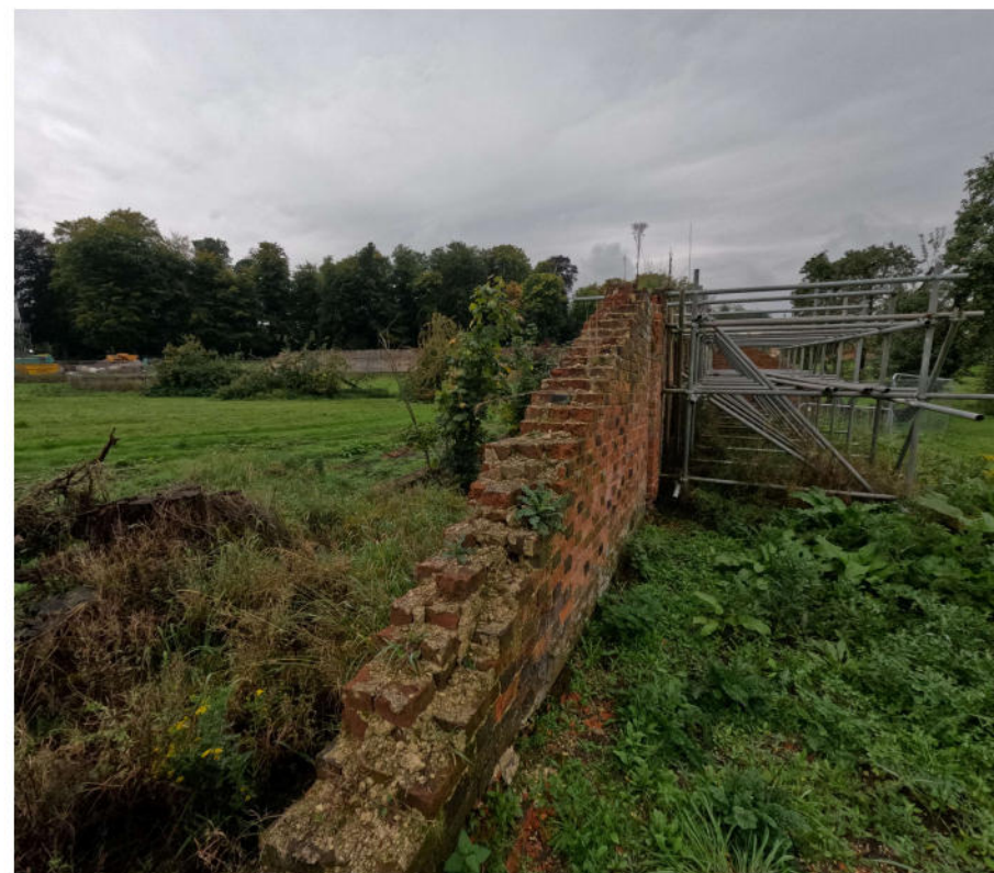
Figure 21 - Existing spine wall brickwork
