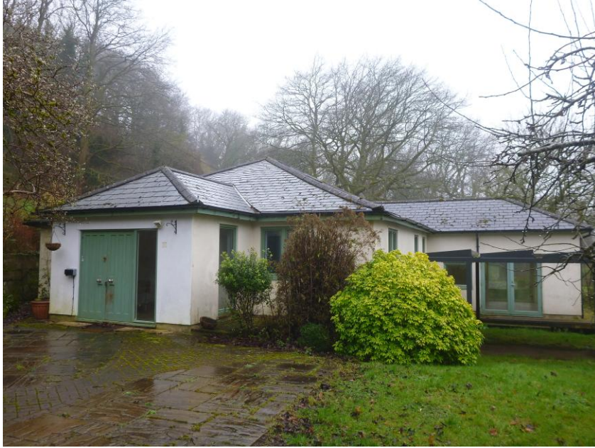
Fig 4: The house at Cleeve Rocks is a single storey property with rendered block walls and a slate roof.
