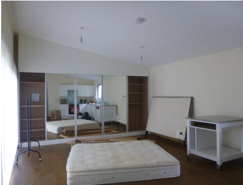
Fig 7: The studio is fully boarded internally, leaving no enclosed void spaces.
