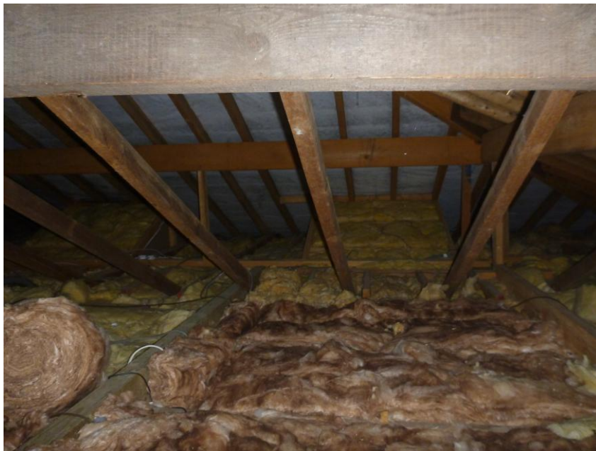
Fig 10: All areas of the loft space of the house were accessible and no evidence of bats was found.
