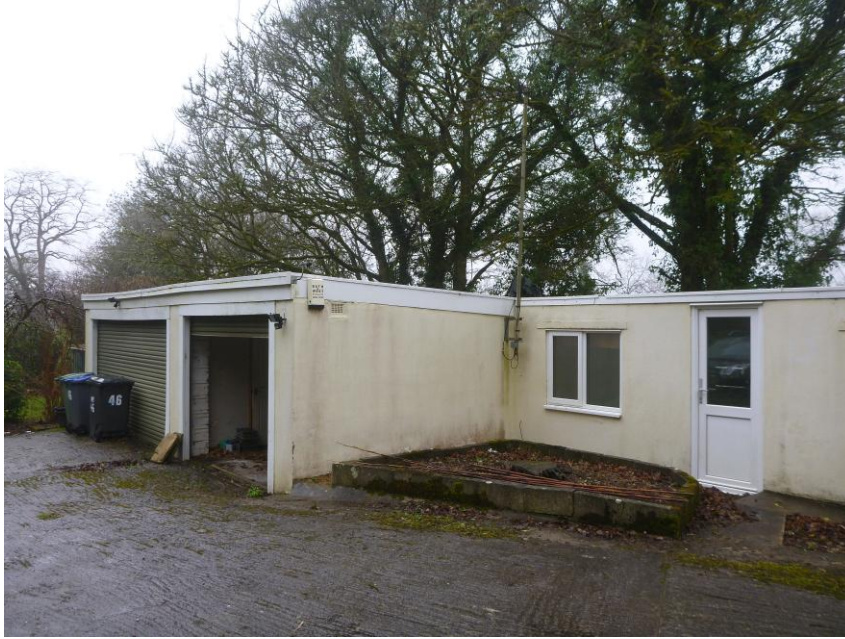
Fig 8: The garage/store/office building at the eastern end of the site.
