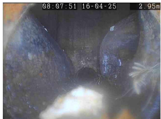
MH2X_32397176-b3e9-44f8-82b6-dda267071c37_20250422_204854_617.jpg, 00:00:55, 2.95 m Roots, fine, finish
