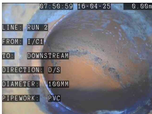
IC1X_b7e59688-eb60-4526-b96a-551b7cd65afd_20250422_203607_555.jpg, 00:00:00, 0.00 m Start node, manhole, reference: IC1
