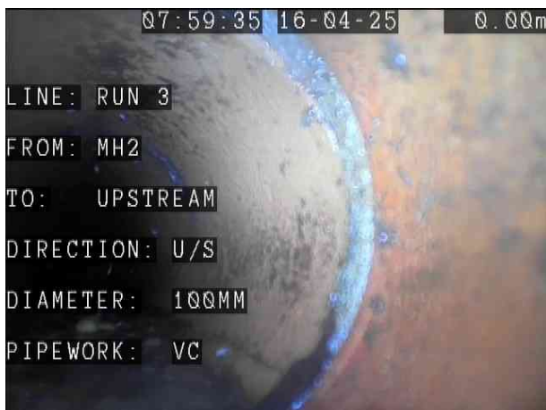
DISUSEDX_699fc097-53f6-46c9-8e3c-40bb3494f093_20250422_204034_192.jpg, 00:00:00, 0.00 m Start node, manhole, reference: MH2
