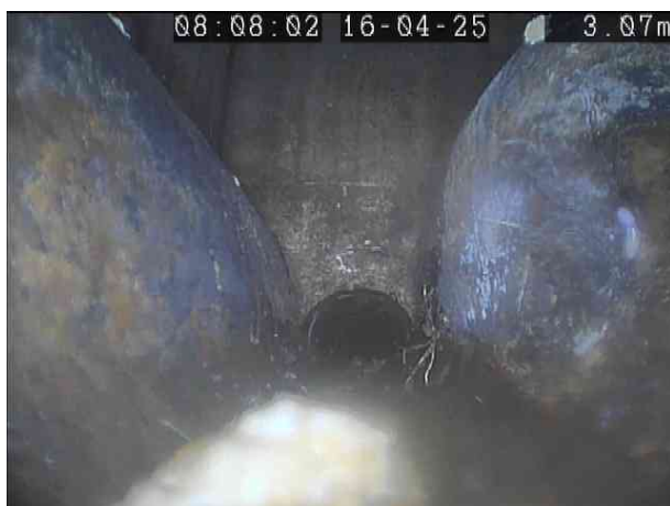
MH2X_9d782177-8fb7-4136-9c76-49fc72d00be8_20250422_204911_766.jpg, 00:01:06, 3.07 m Finish node, manhole, reference: MH3
