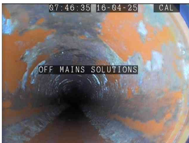
SVP2X_39b73bca-a06f-4ade-8d00-4b345375d709_20250422_202345_311.jpg, 00:00:00, 0.00 m Start node, manhole, reference: IC1
