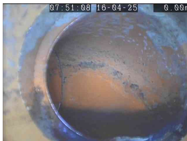
IC1X_7c265984-533b-466f-97b9-df5a4d28b1fc_20250422_203628_469.jpg, 00:00:08, 0.10 m Line deviates left
