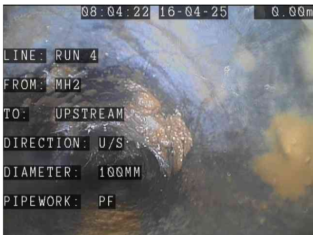
SVP3X_cd49045b-32e7-4a70-832a-121ba95b7b20_20250422_204331_295.jpg, 00:00:00, 0.00 m Start node, manhole, reference: MH2
