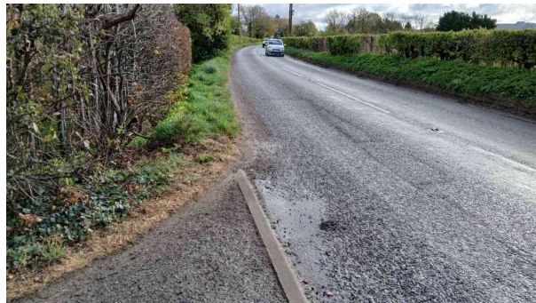
road to front of properties
