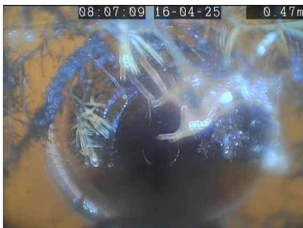
MH2X_93f4c21f-08f1-4a5d-bf7c-08e50e9413d2_20250422_204816_727.jpg, 00:00:14, 0.59 m Roots, fine, start
