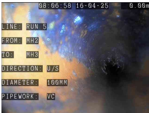
MH2X_937808e8-e1bd-4e08-8414-d06b8045331e_20250422_204646_540.jpg, 00:00:00, 0.00 m Start node, manhole, reference: MH2
