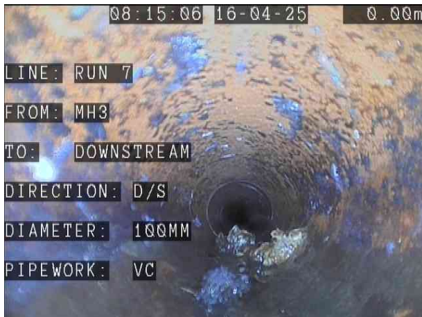
MH3X_eeb99af2-2db1-4137-a4b4-3bfbde2c9ffd_20250422_205733_218.jpg, 00:00:00, 0.00 m Start node, manhole, reference: MH3
