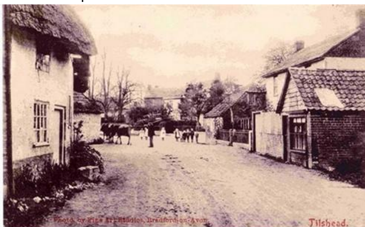
From Tilshead Village website, Primrose Cottage to the left (door now blocked)
