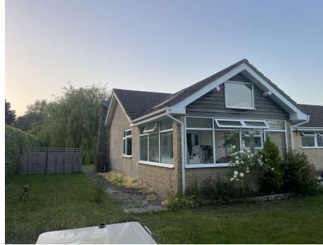
V1 B1-2 surveyor photo
