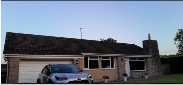
V1 B1-4 surveyor photo
