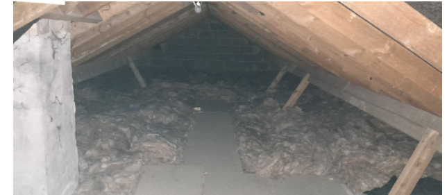
Figure 1a: Loft Void
