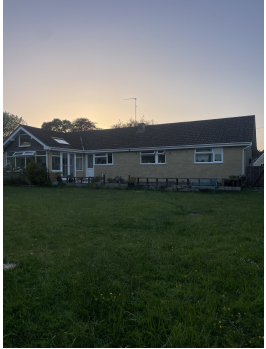
V1 B1-1 surveyor photo
