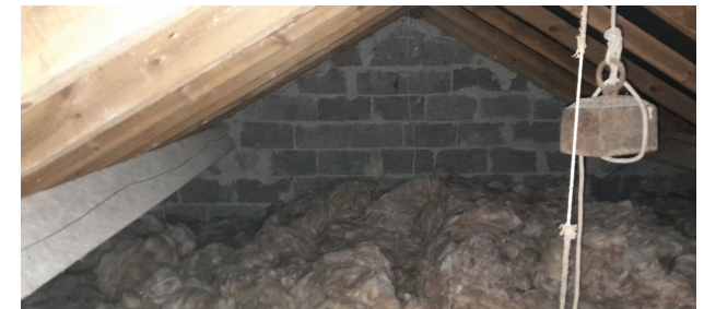
Figure 1b: Loft void
