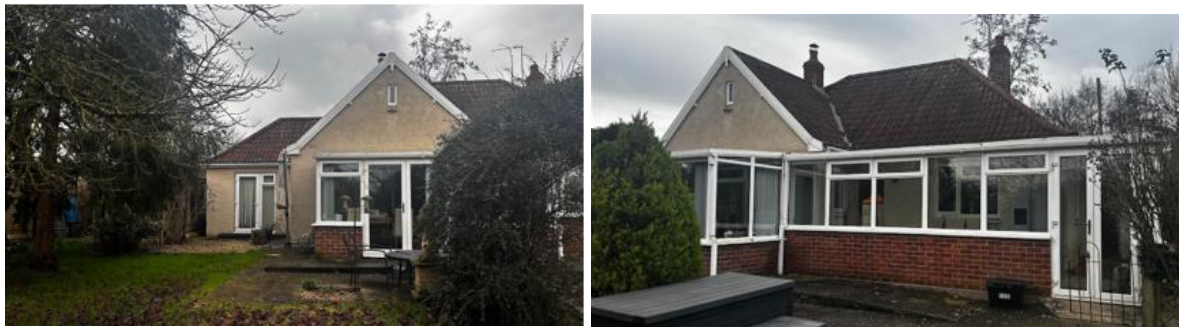
Figure 3: View of the principal south east elevation of the property
