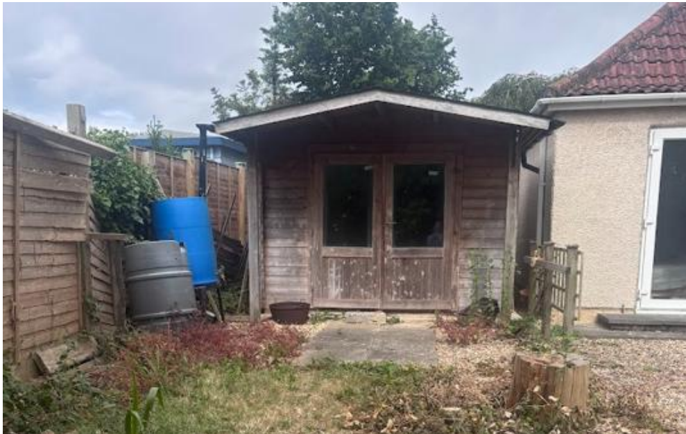
Figure 11: Existing outbuilding to be removed with the proposed extension extending from the existing patio door to the right of the site photo.
