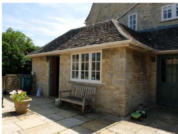
Fig.25 Phipps extension on the NW of the kitchen
