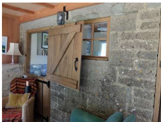
Fig.38 Exposed walls and joinery retains character
