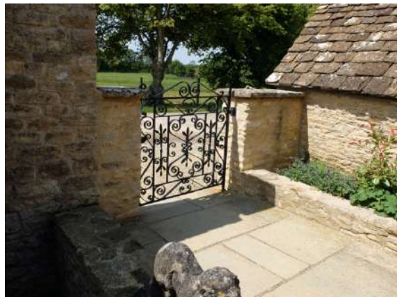
Fig.32 Rebuilt garden wall and new gate to rear courtyard (16)
