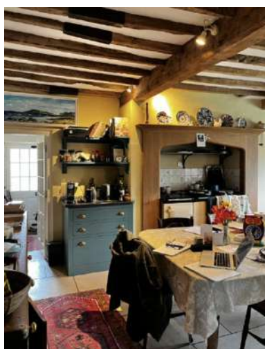
Fig.43 Kitchen removed partition (2)
