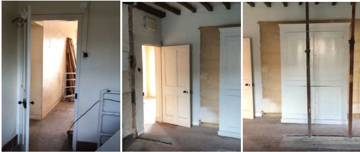
Figs.56 - 61 Kitchen, removed partitions (2) Pantry (3) and Rear Lobby (1)
