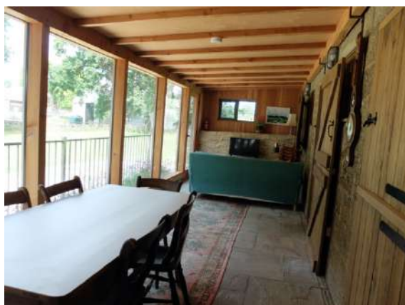
Fig.37 Internal view of the glazed front
