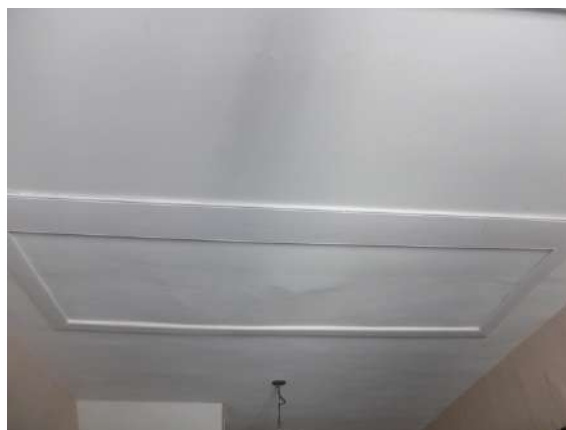
Fig.42 Hatch in ceiling central hallway GF (6)
