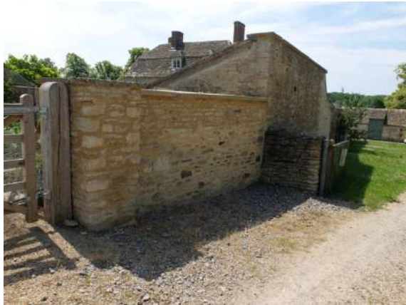
Fig.29 Rebuilt sections of boundary wall (14)
