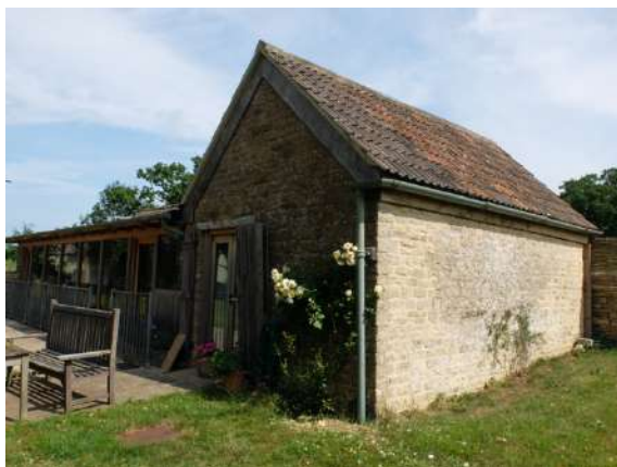
Fig.33 Converted Piggery viewed from the west
