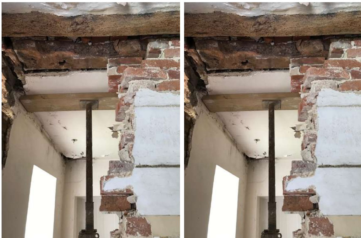
Figs.62 - 63 Removal of Pantry wall revealing joists/beams laid in parallel (kept in situ) and manufactured brick double skin partition.
