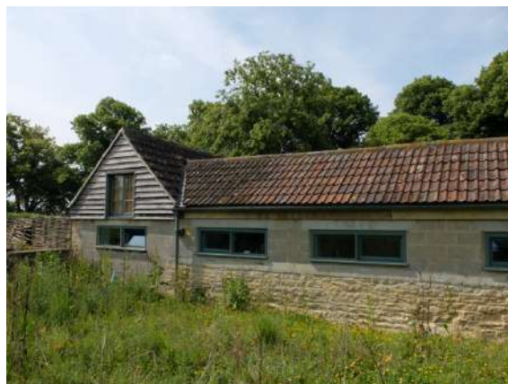
Fig.36 Rear of the Piggery
