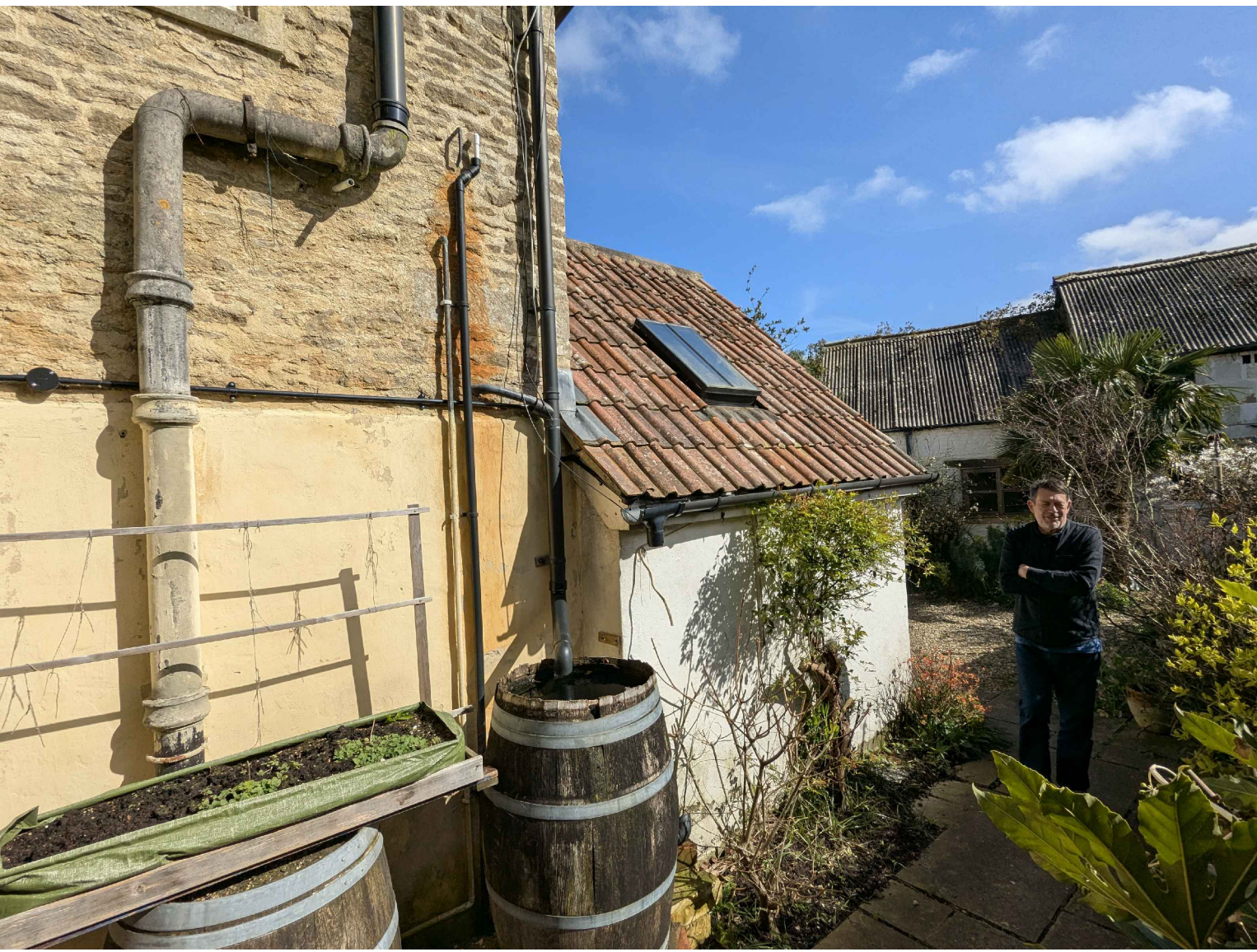
Image: Existing roof light to be replaced is not of conservation style
