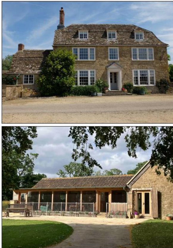
Figure 5 & 6: Recent site images – Principal farmhouse & The Piggery
