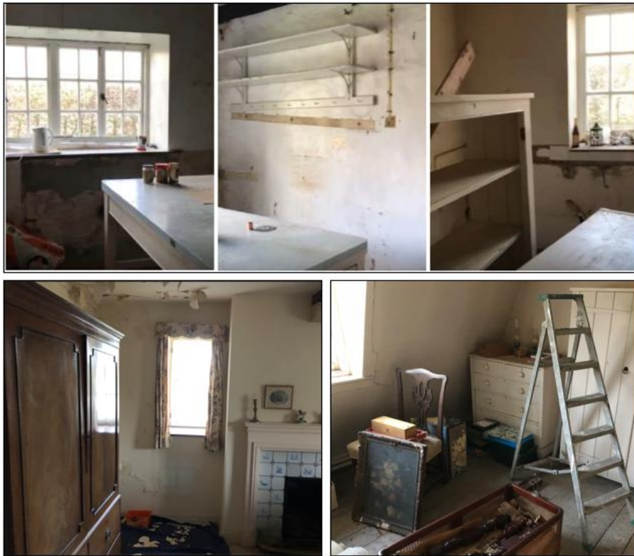
Figure 7: Images of property in advance of renovation
