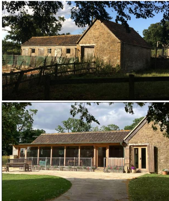
Figure 10 & 11: Before conversion & recent image of The Piggery
