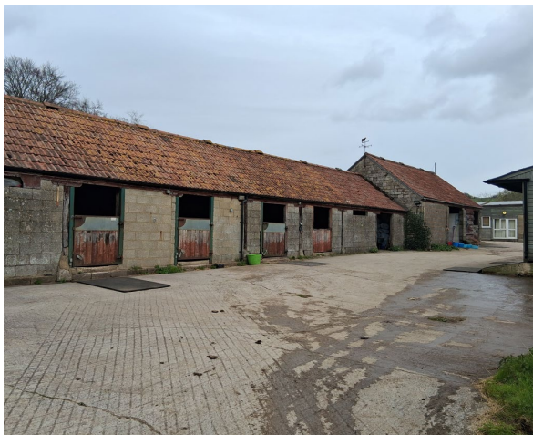
Fig 9: General view of former cowshed with stable to the right
