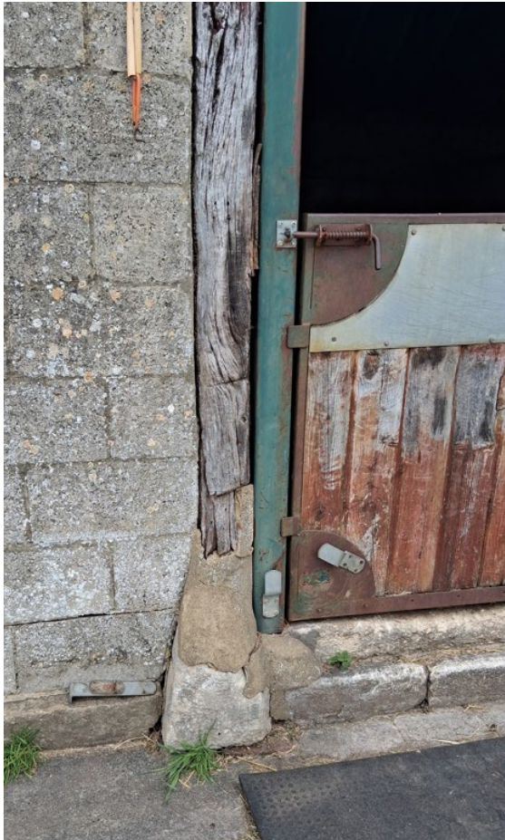
Fig 20: detail of vertical timber post on staddle stone, blockwork infill and modern stable doors.
