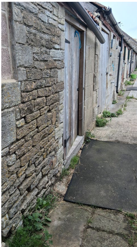
Fig 12: Rubblestone wall to feed store
