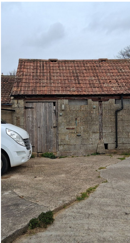
Fig 17: Junction between former cowshed & feed store
