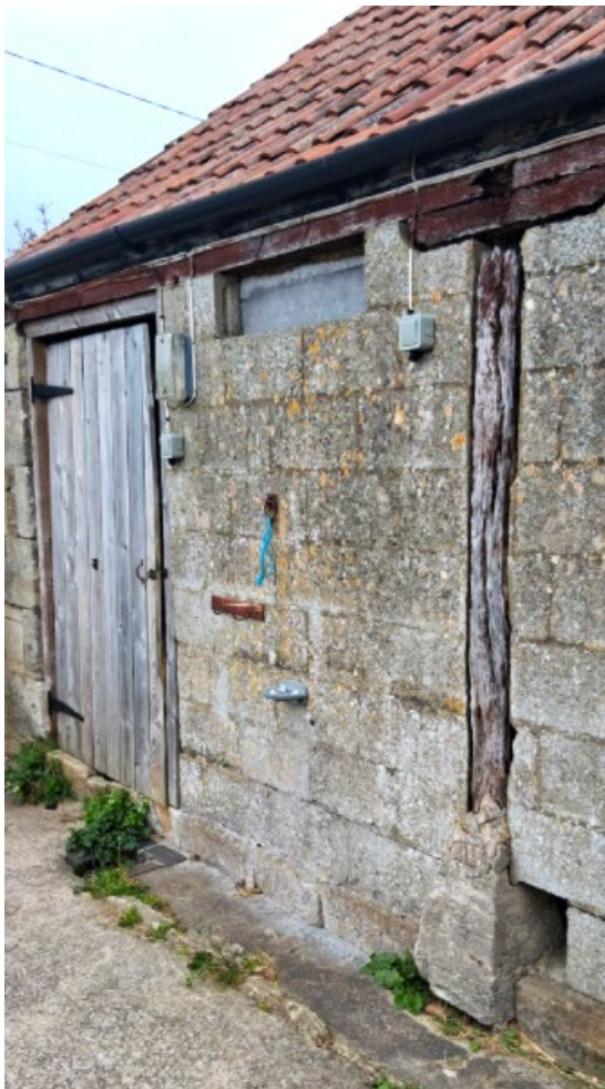
Fig 10: Timber post on staddle stone
