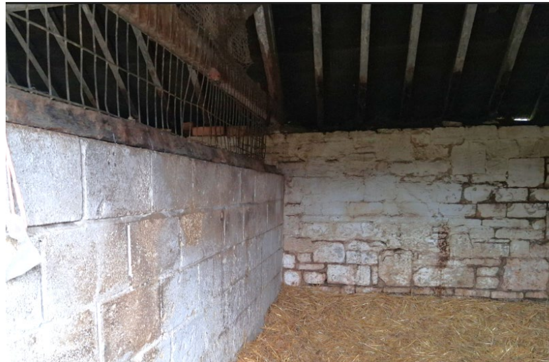
Fig 14: Modern breezeblock dividing walls between stables
