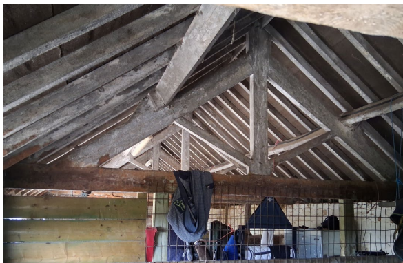
Fig 8: King-post roof trusses
