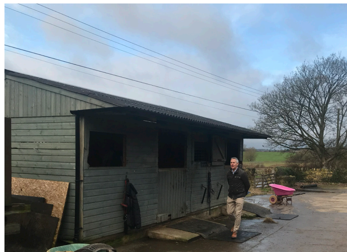
Fig 4 Temporary timber stable to be removed
