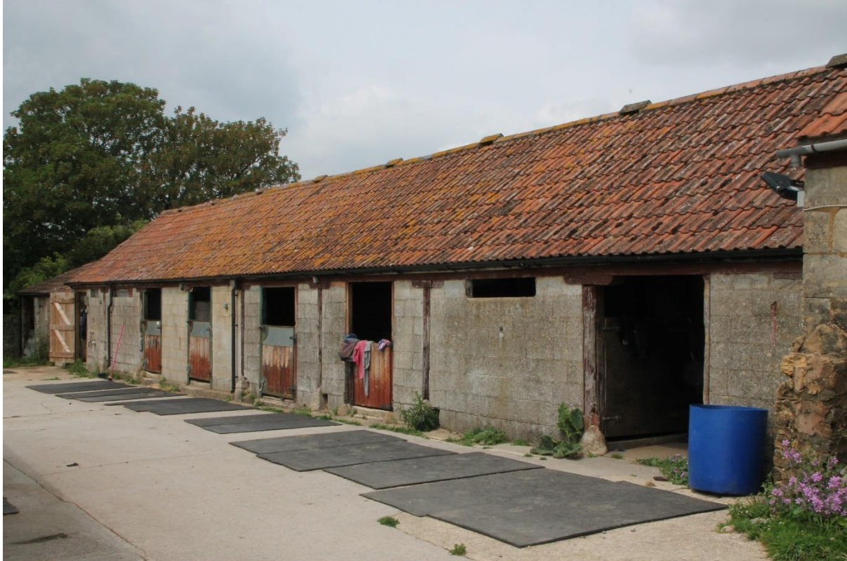
Photograph 4: showing a view of Building 1
