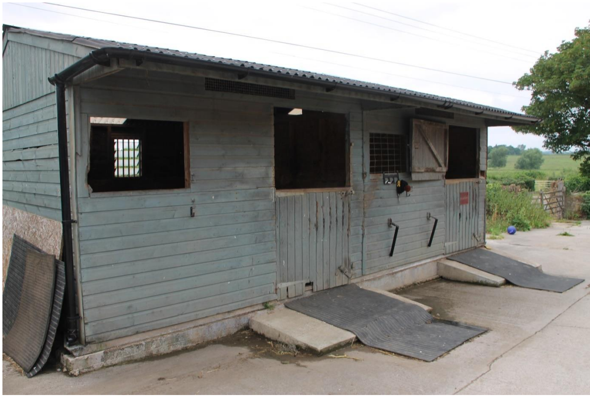
Photograph 6: showing a view of Building 2
