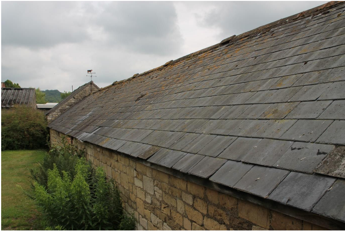
Photograph 5: showing a view of the rear (northern) view of Building 1
