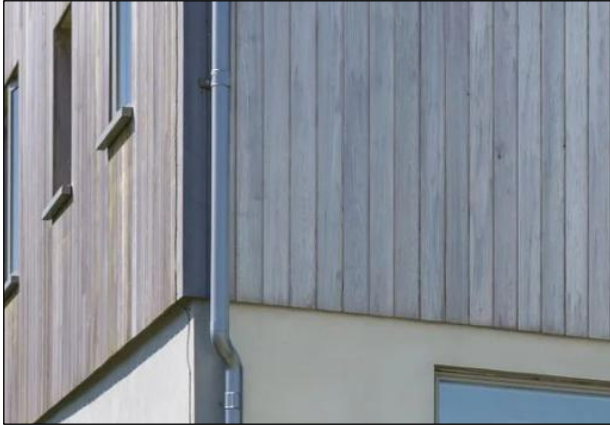
Examples of larch vertical cladding
