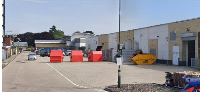
Image shows rear of units in servicing area, housing plant, bin stores, access for loading and delivery.
