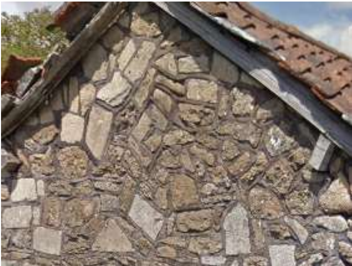
Existing Materials; Rubble stone and clay pan-tile roof.
