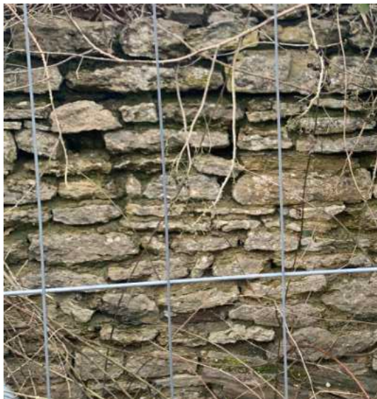
Reclaimed stone from existing barn building to be used in the retail unit construction.
