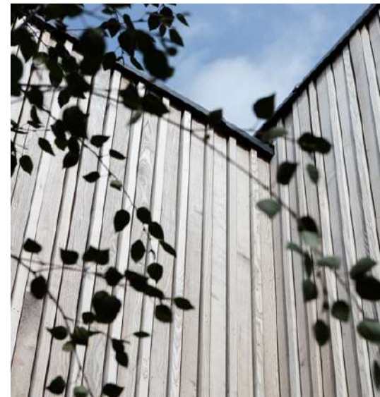
Articulated Cladding - Allowed to weather and silver.
