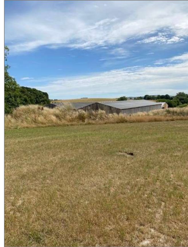
Figure 3: View southeast from the site across existing agricultural barns
