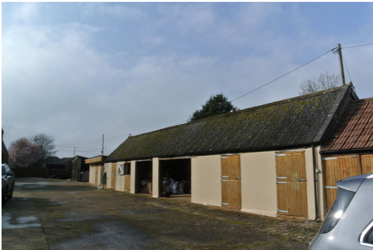
Photograph 1: showing external view of the target building (facing north-west)
