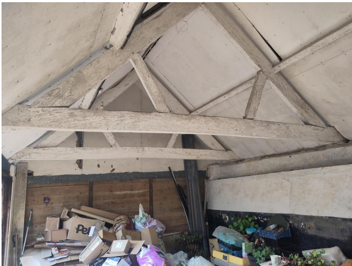
Photograph 2: showing an internal view of the target building (facing west)
